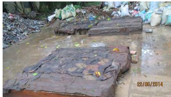
Figure: 3.20 Curing of Beams
