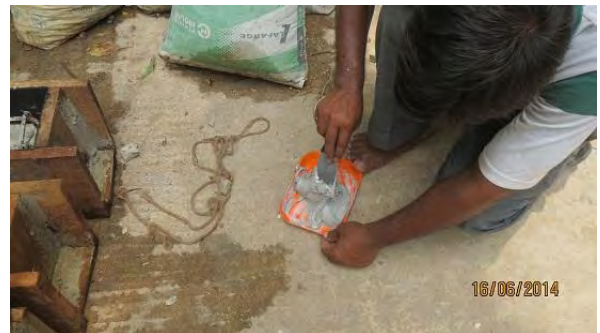
Figure: 3.15 75MPa Epoxy Preparation
