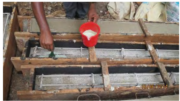
Figure: 3.13 Application of 50MPa Epoxy
