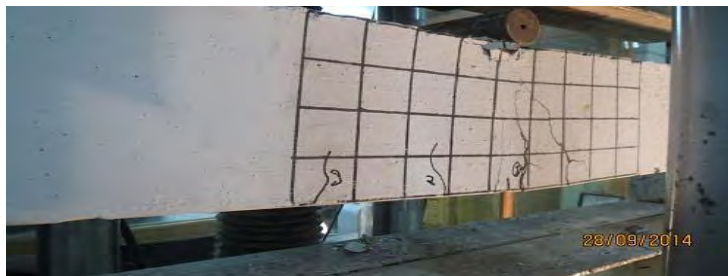
Figure 4.1 Failure Pattern of Specimen-FB3
