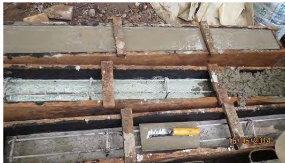
Figure: 3.14 After 50MPa Epoxy Application Beam Casting
