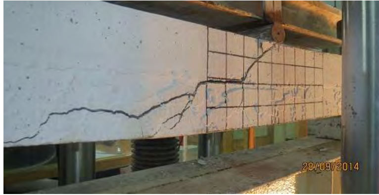
Figure 4.28 Failure Pattern of Specimen-HB57C
