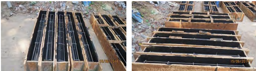
Figure: 3.8 Formwork Ready for Casting. Reinforcements Were Kept In Formwork
