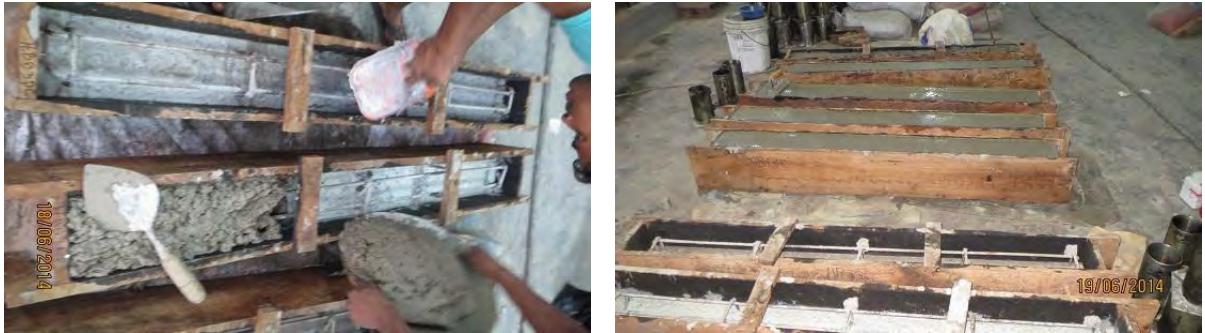
Figure: 3.19 After Application of Bonding Agent Beam Casting
