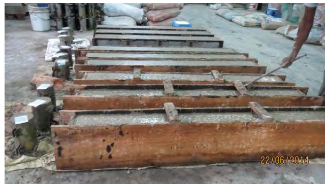
Figure .3.21 Casting of Last Nine Beam Specimens
