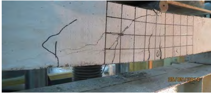
Figure 4.22 Failure Pattern of Specimen-HB51C
