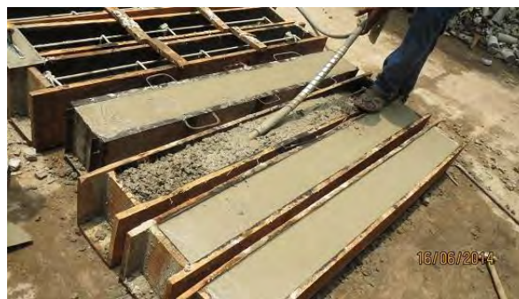
Figure: 3.17 After Application Of 75MPa Epoxy Half Prepared Beams Were Vibrated and Cast
