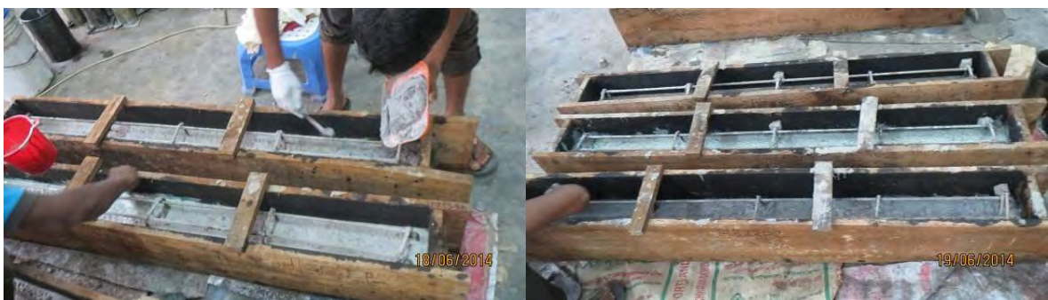
Figure: 3.18 Application of 75MPa Epoxy And 50MPa Epoxy After Three Days
