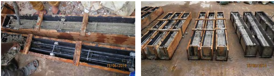
Figure: 3.9 Concrete Was Poured In The Formwork
