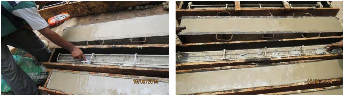
Figure: 3.16 Application of 75MPa Epoxy
