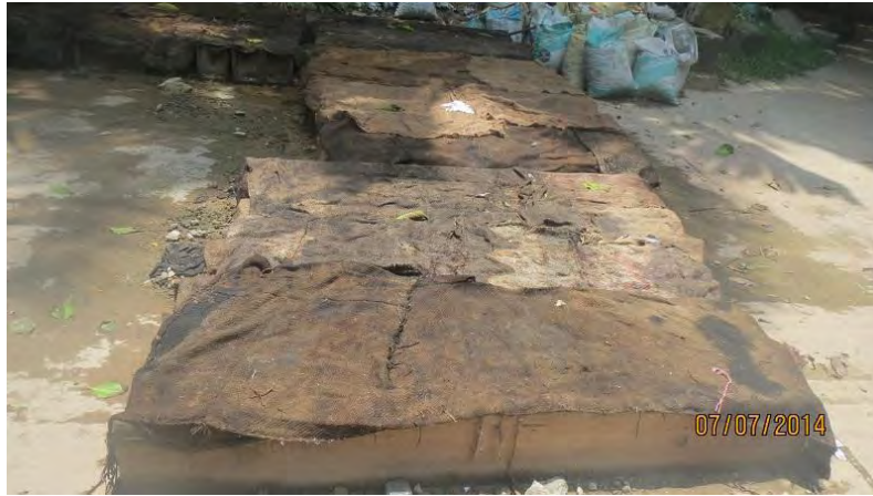
Figure: 3.22 Curing of All Thirty Beams
