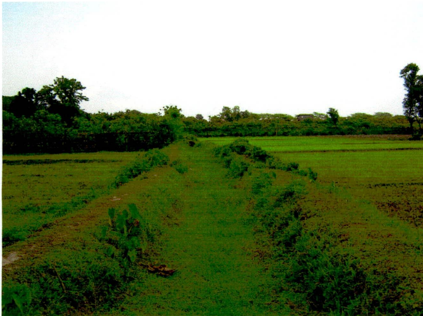
Fig.3.8: A view of unlined field channel in MDIP
