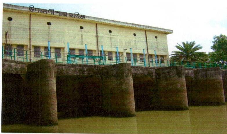
Fig. 3.4: A view of Udhamdi Pump House in MDIP
