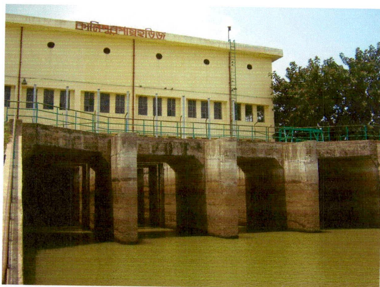
Fig. 3.5: A view of Kalipur Pump House in MDIP
