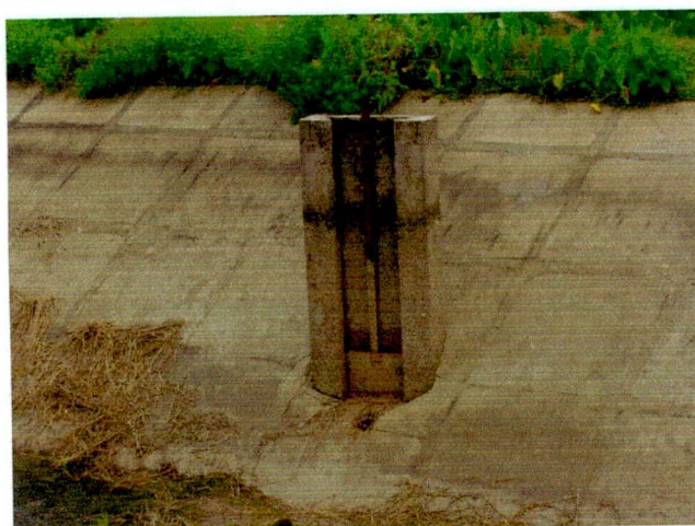
Fig. 3.6: A View of Newly Constructed Turnout in MDIP
