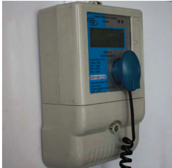
Figure A 2.3: Optical Meter Reader Attached With Digital Energy Meter
