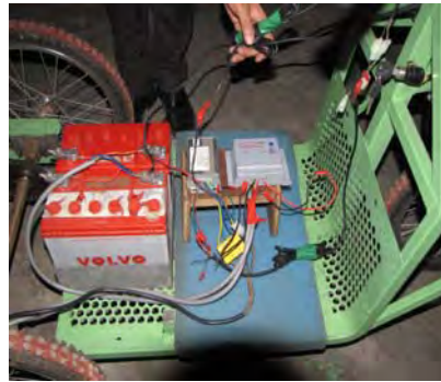
Figure 4.33(a): Battery system with controller.
