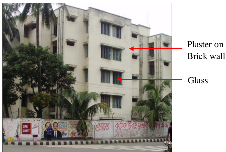
Figure 3.25 Different types of building materials used in Road Junction 3 - Shahid Minar Road (Photo credit: Self)
