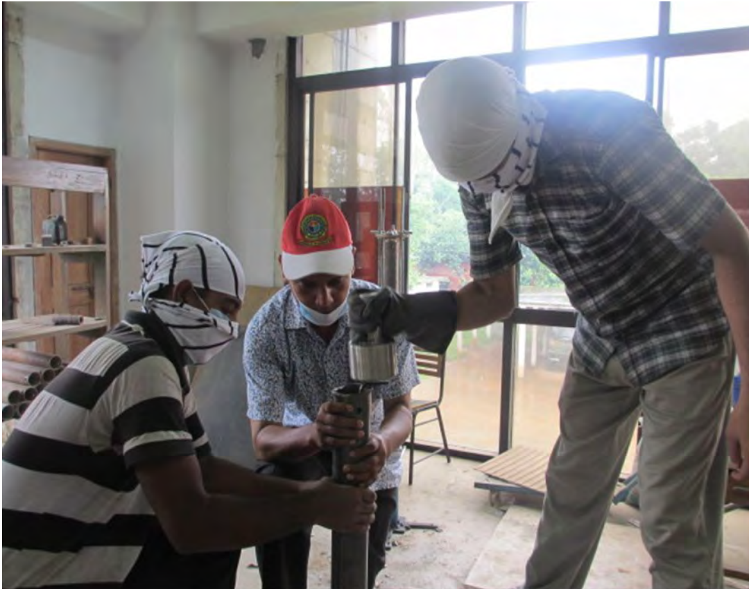
Figure 3.13 (f): Compacting the SCP Sand
