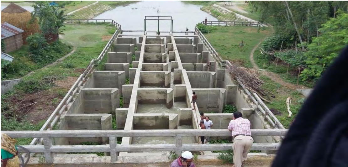
Figure 2.2: Sariakandi fish pass (view towards Bangali River)
