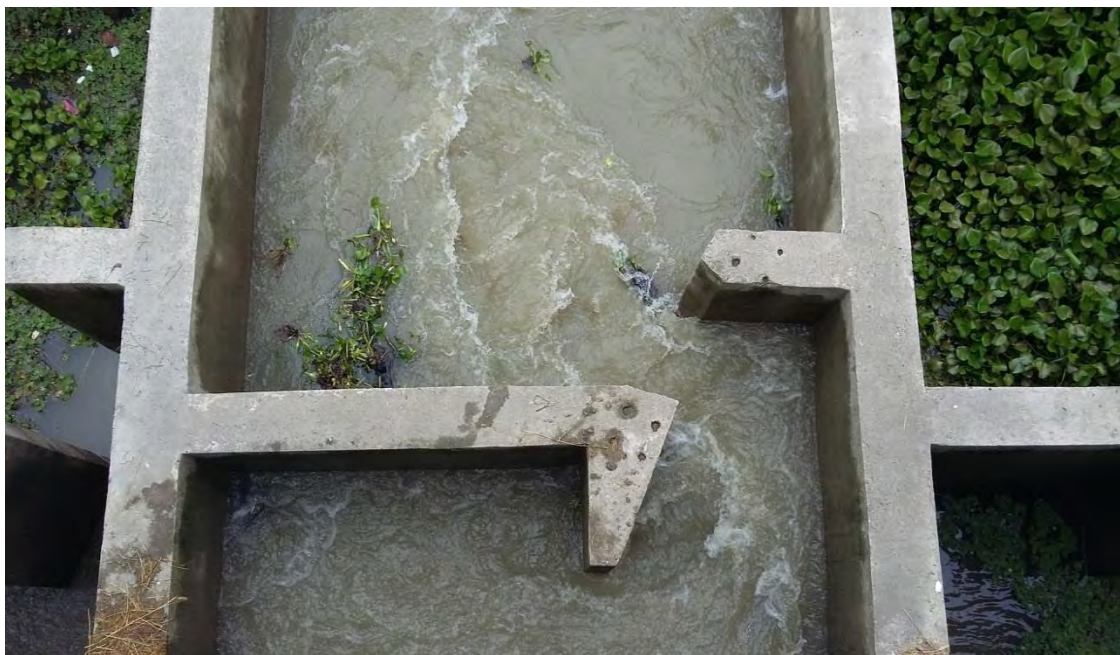
Figure 2.4: Flow pattern at the opening of a pool of Sariakandi fish pass
