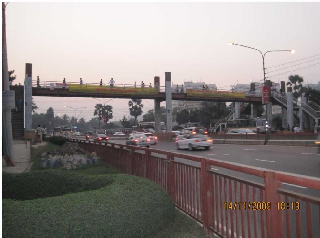
Figure 1.6: Footbridge near Radisson Water Garden Hotel over Airport road.
