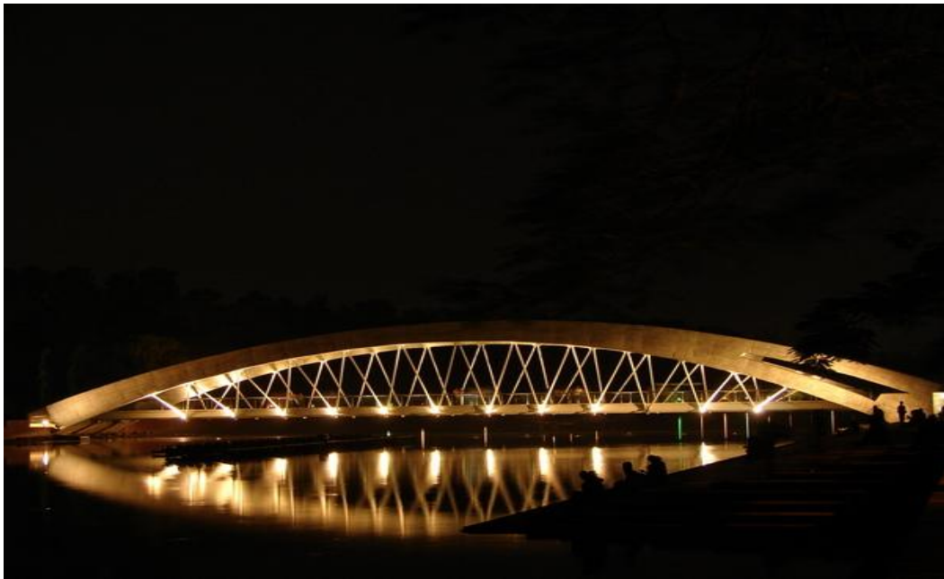
Figure 1.3: Footbridge over the Crescent Lake in Dhaka.
