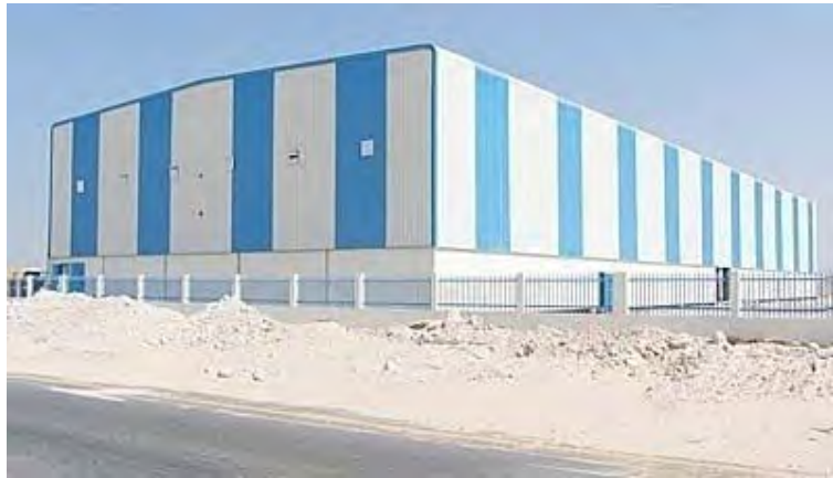
Figure 1.4: Trapezoidal through fixed Aluminium composite panel for façade cladding Versacor Ultima
