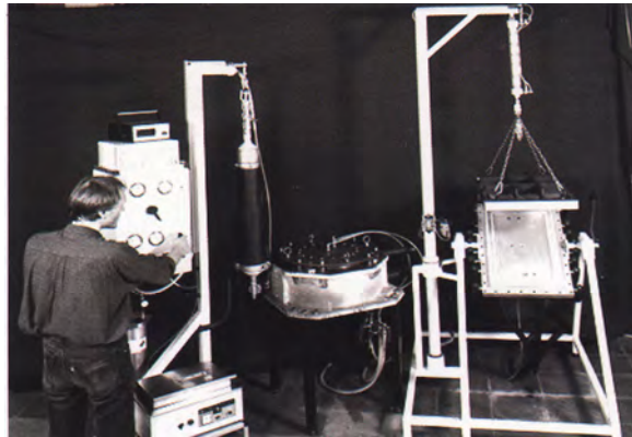
Figure 3.11: Resin Transfer Moulding (RTM).
