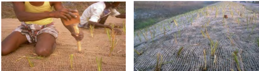
Figure 4.35 Vetiver plantation at embankment slope: plantation procedure and newly planted vetiver (right)
