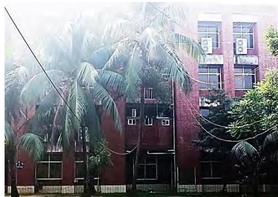
Figure 4.28: Front View of Building No.9D
