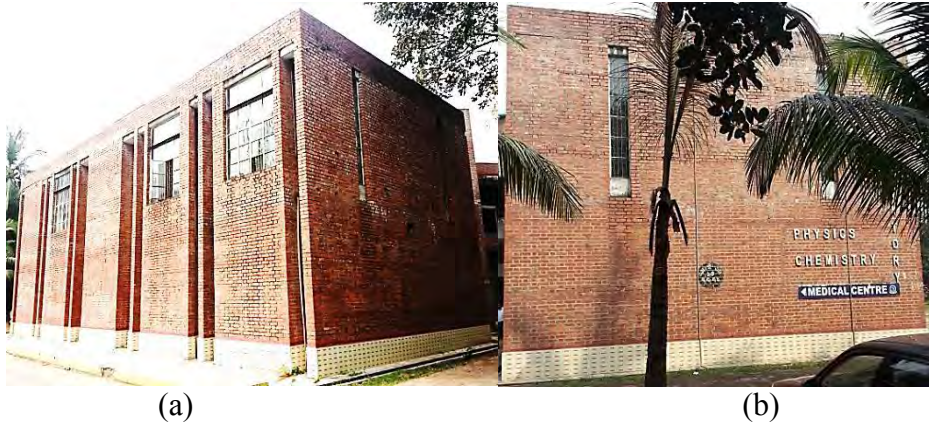
Figure 4.16: (a) Front View and (b) Side View of Building No.15A
