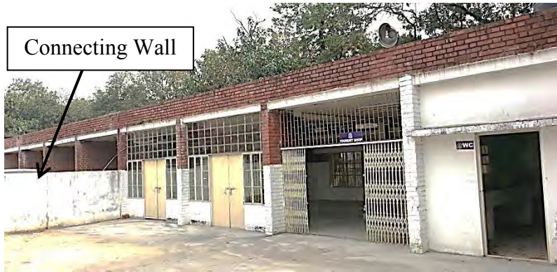
Figure 4.4: Front View of Building No. 6B
