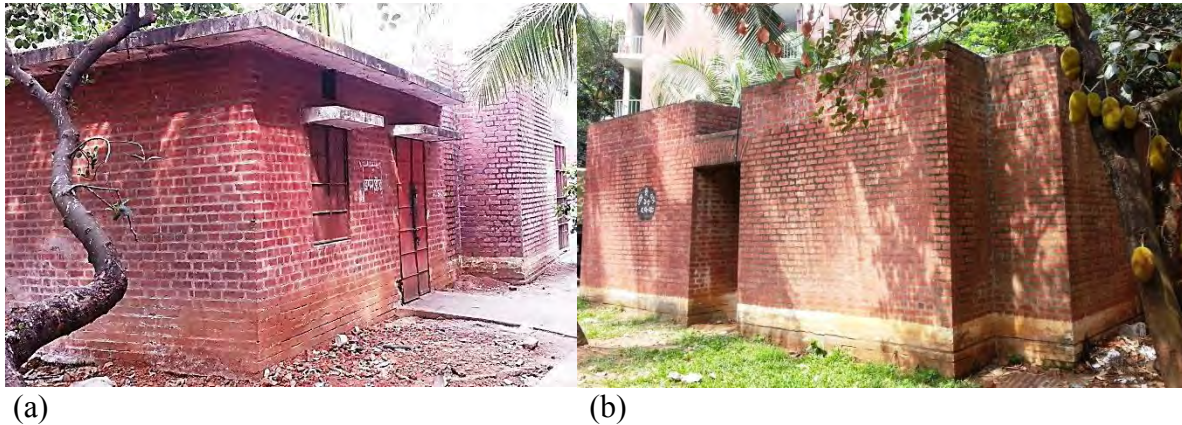
Figure 4.10: (a) Front and (b) Side View of Building No. 13
