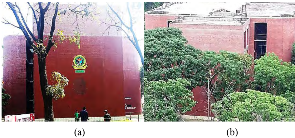
Figure 4.27: (a) Front View and (b) Side View of Building No.9A
