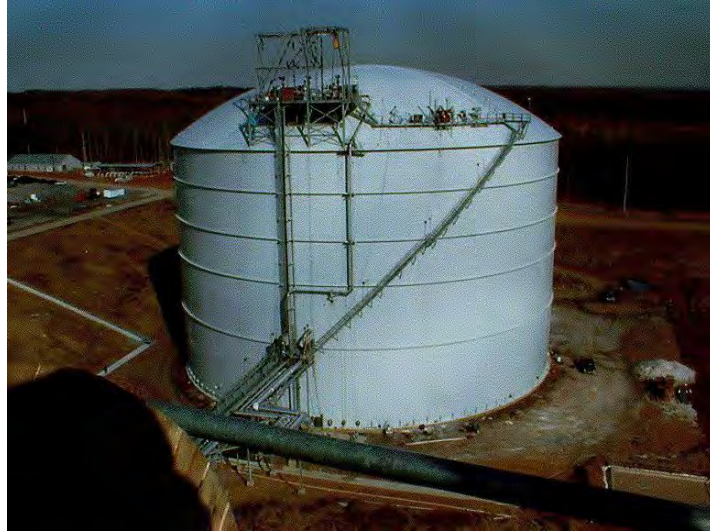
Figure 3.3: LNG storage tank (Source: Federal Energy Regulatory Commission)
