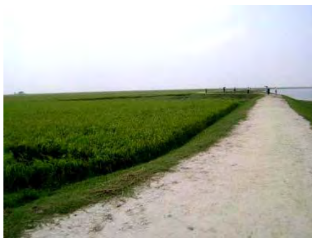
Figure 3: Submersible embankment protecting Boro paddy
