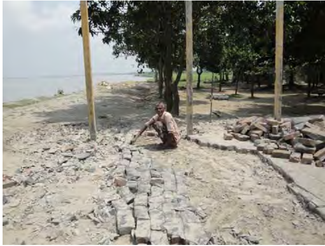
Fig C10: School shifting from bankside on 1 st June 2010
