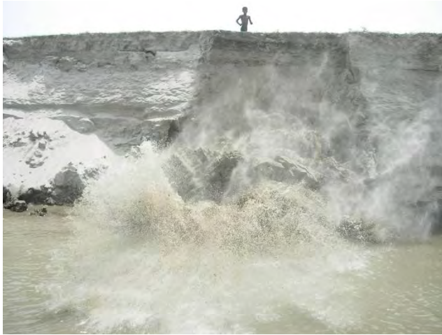
Fig C1: Sudden bank failure on 23 rd April 2010
