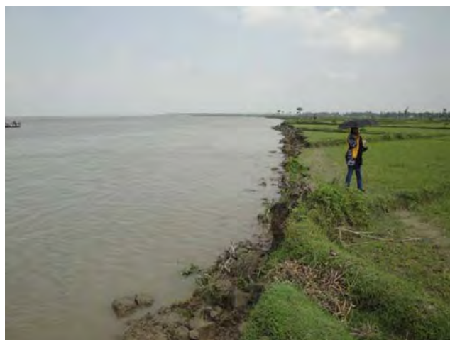
Fig C6: Bankline survey on 1 st June 2010
