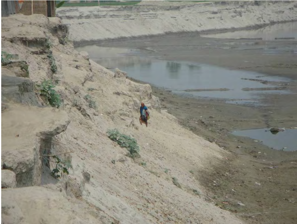
Figure 6.12: Difficulty to go through the steep slope
