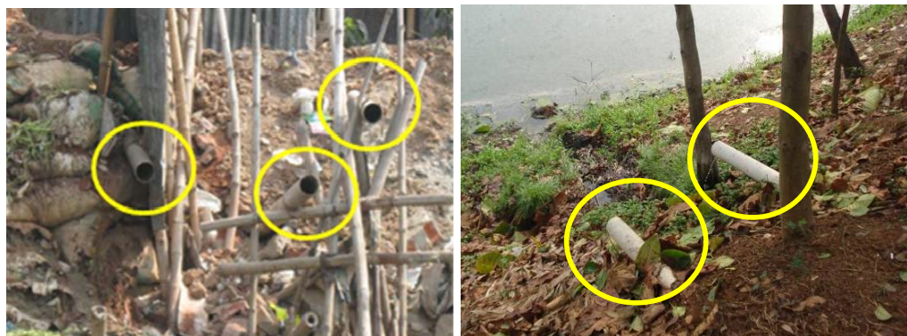
(a) (b) Fig 3.4: Private Outfalls, (a) from a construction site near Outfall ID#105 and (b) from a parking lot near R#96
