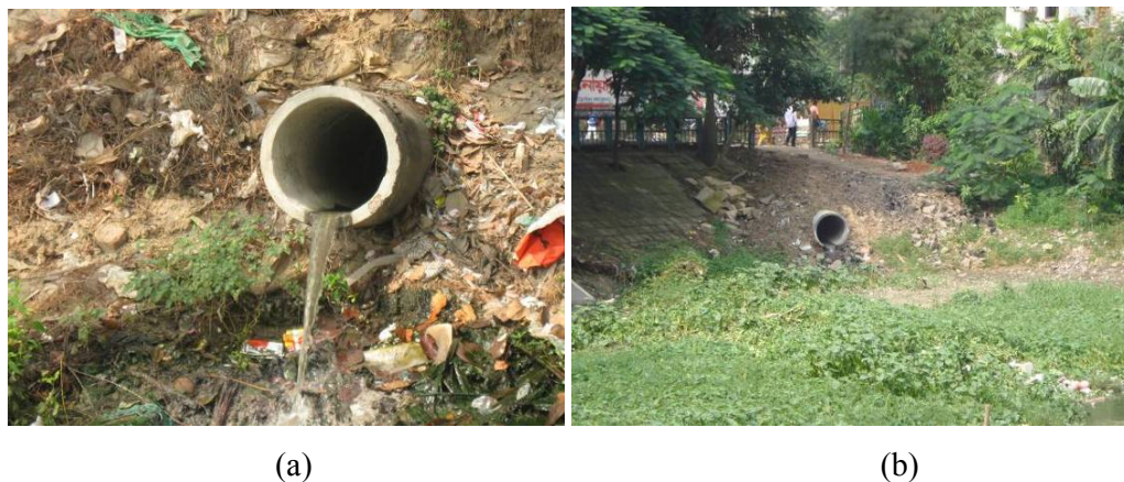
Fig 3.1: Pipe outfalls, (a) near R#136 and (b) near Baridhara DOHS
