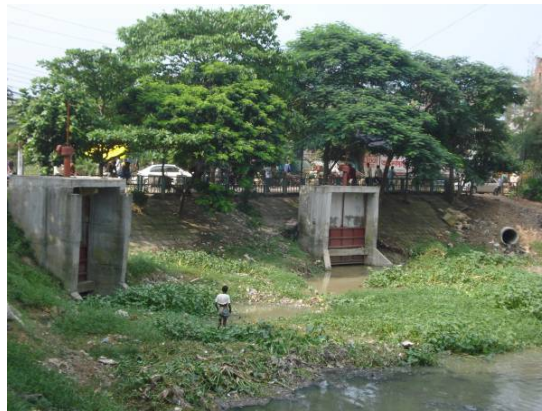
Fig 3.3: Box culverts discharging into Gulshan Lake near Baridhara DOHS
