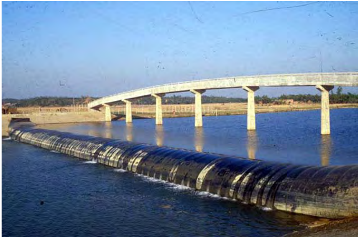
Figure 2.3: Bakkhali rubber dam, Cox's Bazaar.
