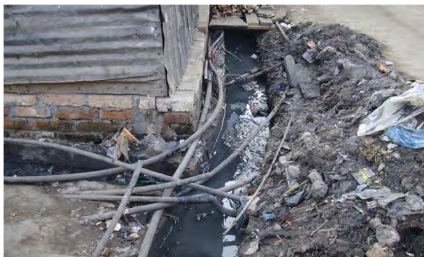
Figure 5.3: Water Pipes Remains in Drain
