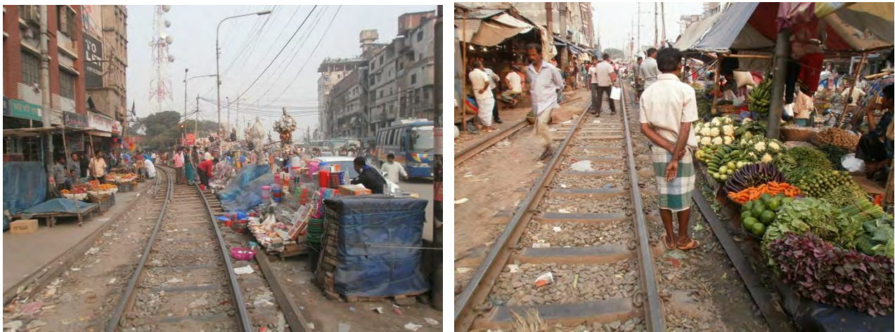
Plate No. 01: Railway land is occupied by (i) wayside bazaars, small vendors, slums and (ii) buildings leaving very little space beside the tracks for safe movement of trains. (Narayanganj ) Source: Author
