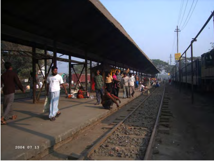
Plate 07: Low and shanty Platform of Narayanganj Railway Station.
