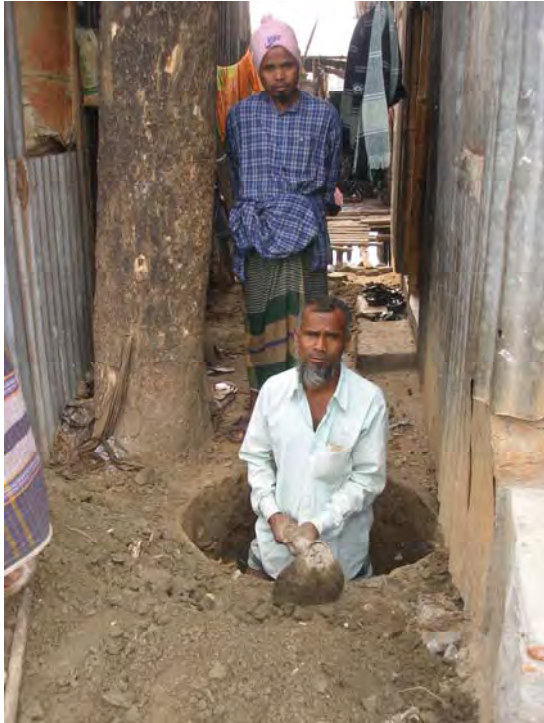
Plate 6.7 : Practical instruction for construction of sanitary latrine, (date 07/08/2007), Source ARBAN
