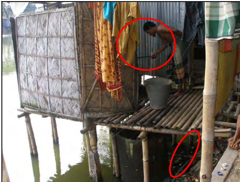
Plate 4.2: Piped water supply used by installing hand tube-well, households at the edge of pond
