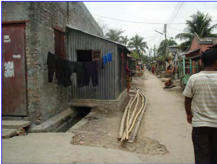
Plate 4.7: Most of the roads are poorly managed in Bauniabandh. Households have encroached the road & drain
