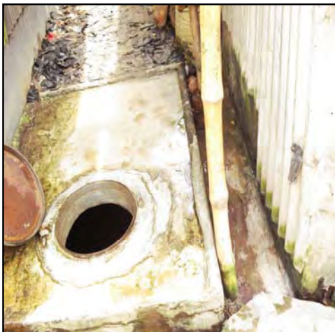
Plate 7.3: The water reservoir located on the walk way
