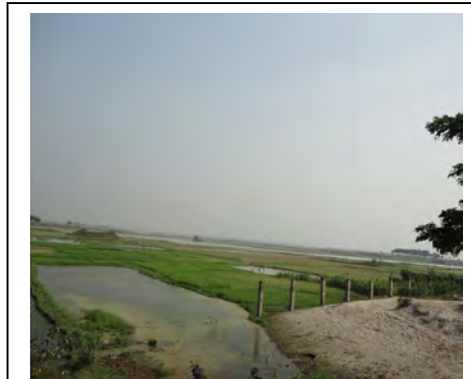
Photograph 4.16: Land filling process
