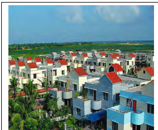
Photograph 4.18: Present project condition
