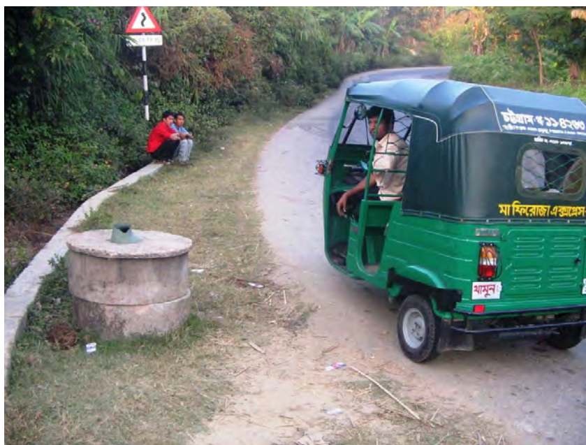
Photo 9.3. Rings slab of a house is left on the boot bottom of a hill
