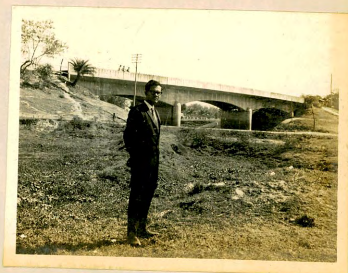
Plate 5.1 Tongi Bridge (The general view showing the spans, girders, etc)
