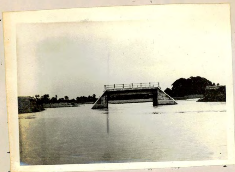
Plate 6.5 Failure due to insufficiency of water-way (The approaches were washed away)
