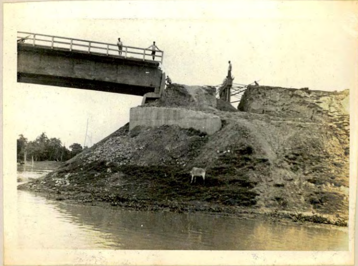
Plate 6.1. A Bhangaghat Bridge (Extra shore-span under construction)
