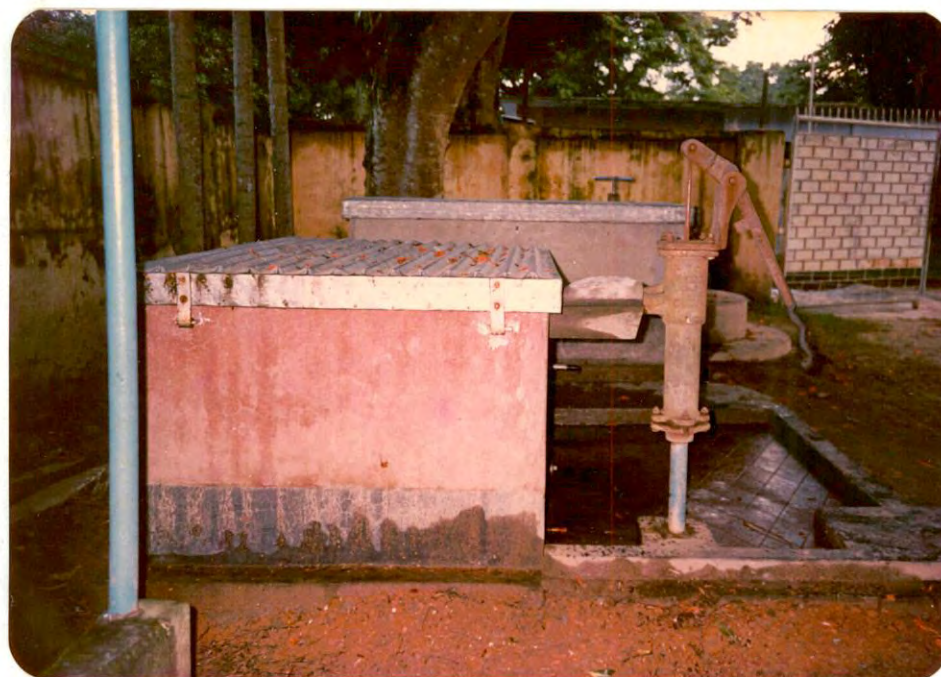
Plate 3.2 Side view of the existing plant at Sirajgonj.
