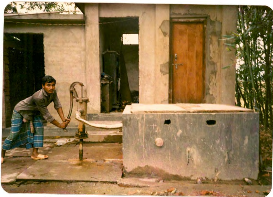
Plate 4.4 Side view of further modified plant
