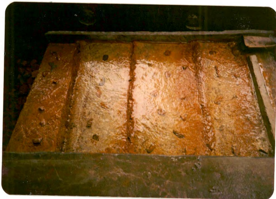
Plate 4.6 Raw water flowover the aeration plate
