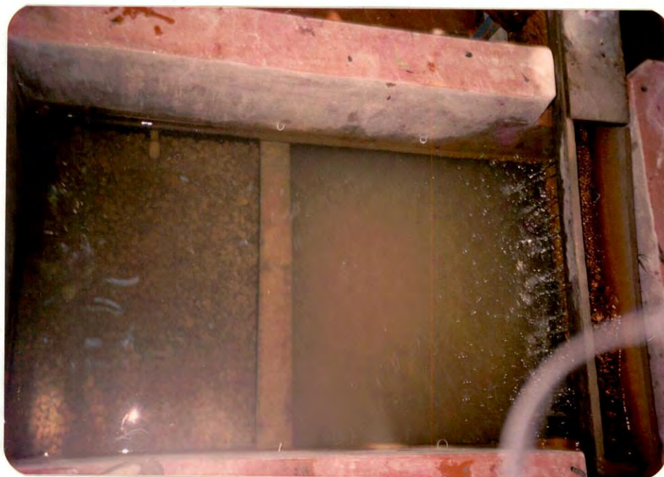
Plate 3.1 Top view of existing iron removal plant.
