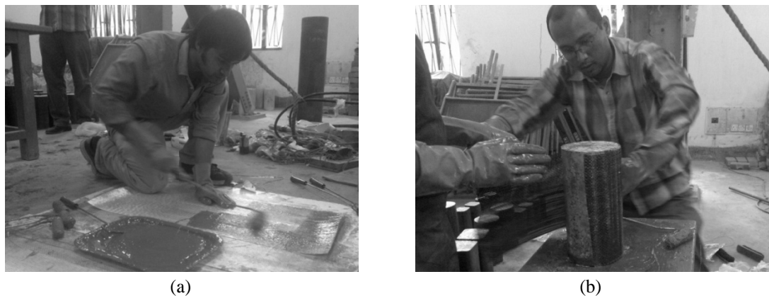
Figure 4.13: Preparation of primer (a) Mixing of Part A and B of primer; thickening for prime coat application with a mechanical mixer operating at 500 rpm at 3 minutes, (b) application of primers on the columns, (c) primer coated columns (surface are darkened by the prime coat)
