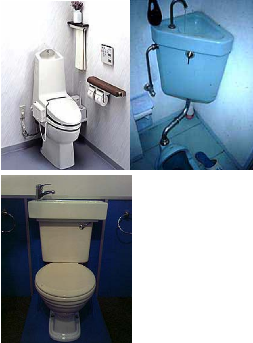
Fig. 2.13 The cistern of this toilet is filled by grey water from the sink above it.
