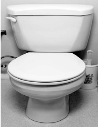
Fig. 2.12 Low-flush toilets, like the 1.33 (US1.6 gpf) model pictured below, are required in all new construction
