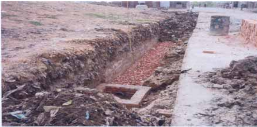
Figure 2.9: Boundary Lechate Drainage System under Construction (BRTC, 2008)
