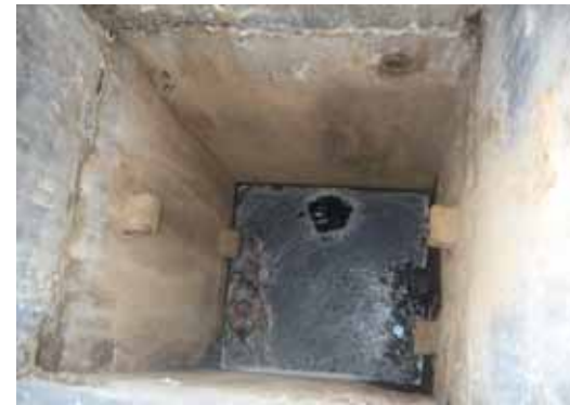
Boundary pipe under submerged condition
