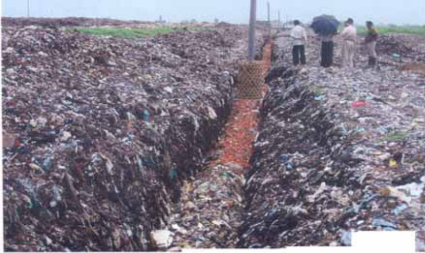
Figure 2.11: Semi-Aerobic System under Construction (BRTC, 2008)
