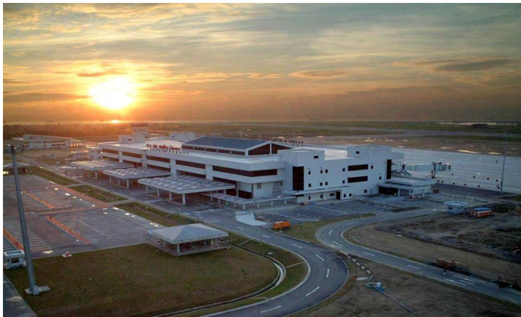
Figure 5.1: Aerial View of Shah Amanat International Airport, Chittagong.
