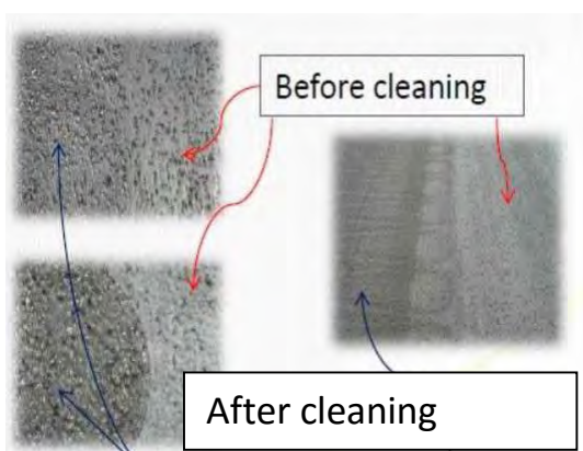
Figure 2.7(a): Before and after cleaning high pressure by water jet
