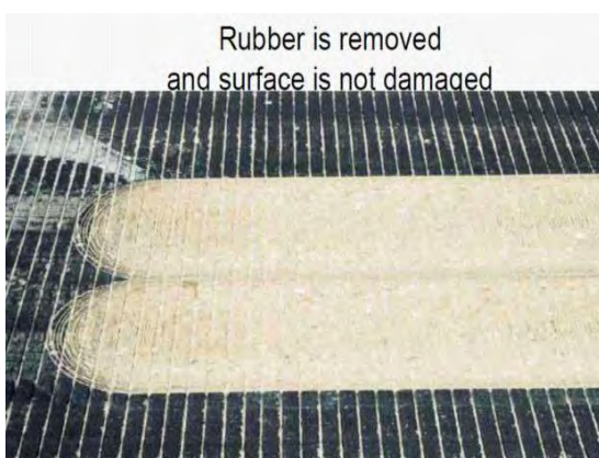
Figure 2.7(c): Cleaning without high pressure damaging surface
