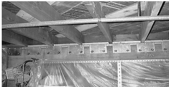
Figure 2.5: Bolted Steel plates to the affected areas.
