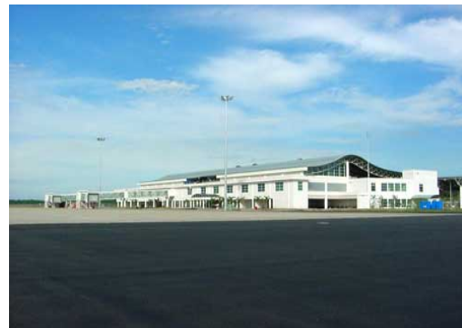
Figure 2.4: PMB in Kuala Lumpur Airport
