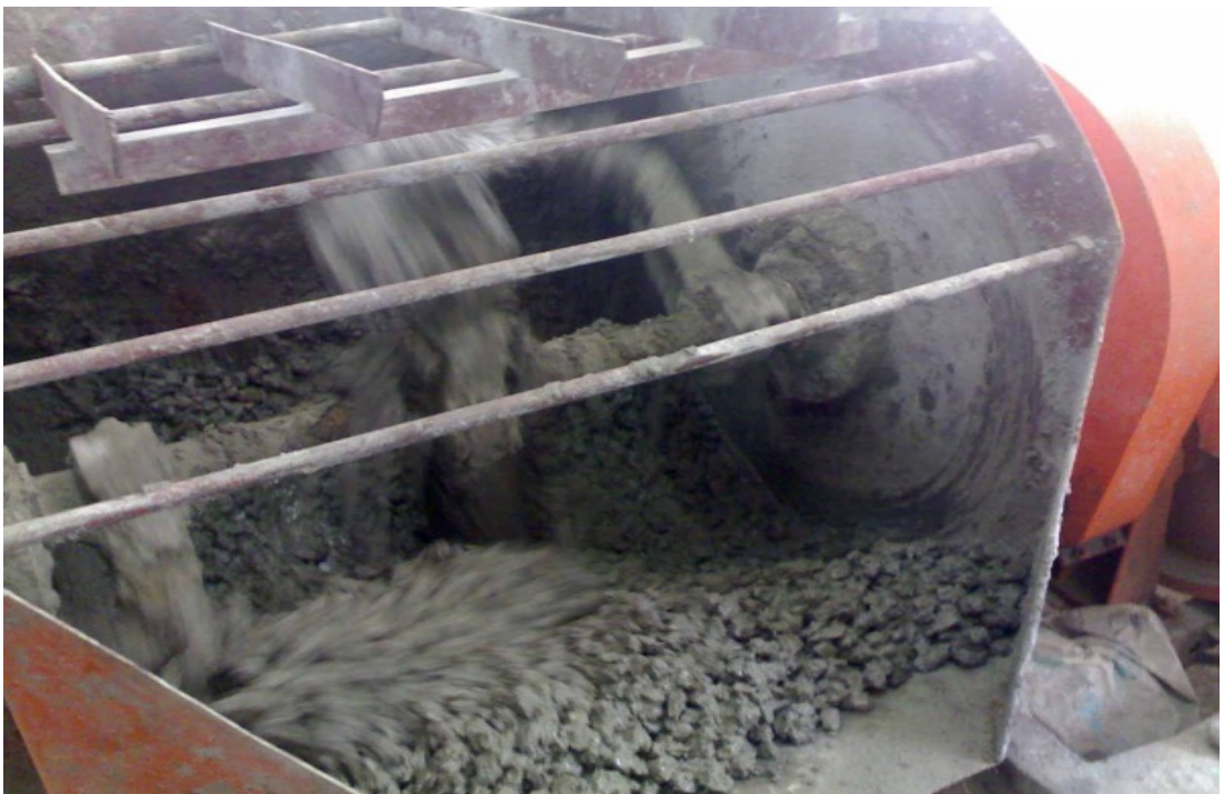
Fig.3.5: Mixing of concrete
