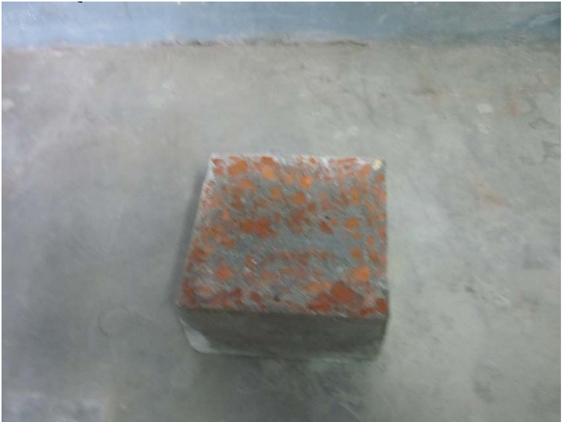
Fig-A8: Wet surface (brick aggregate concrete)
