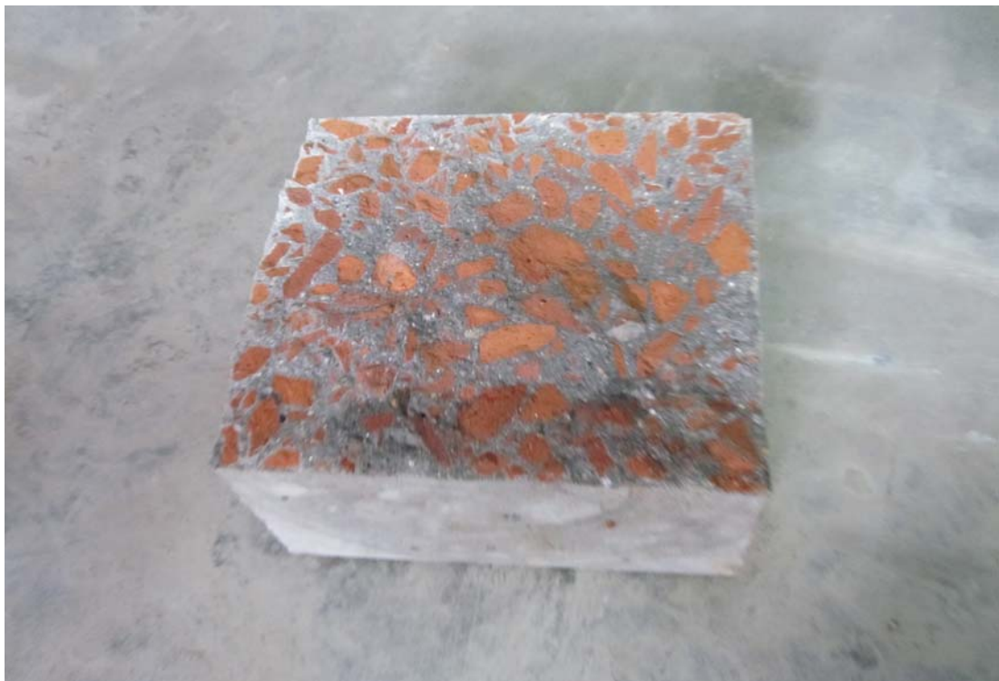
Fig-A2: Wet surface (brick aggregate concrete)
