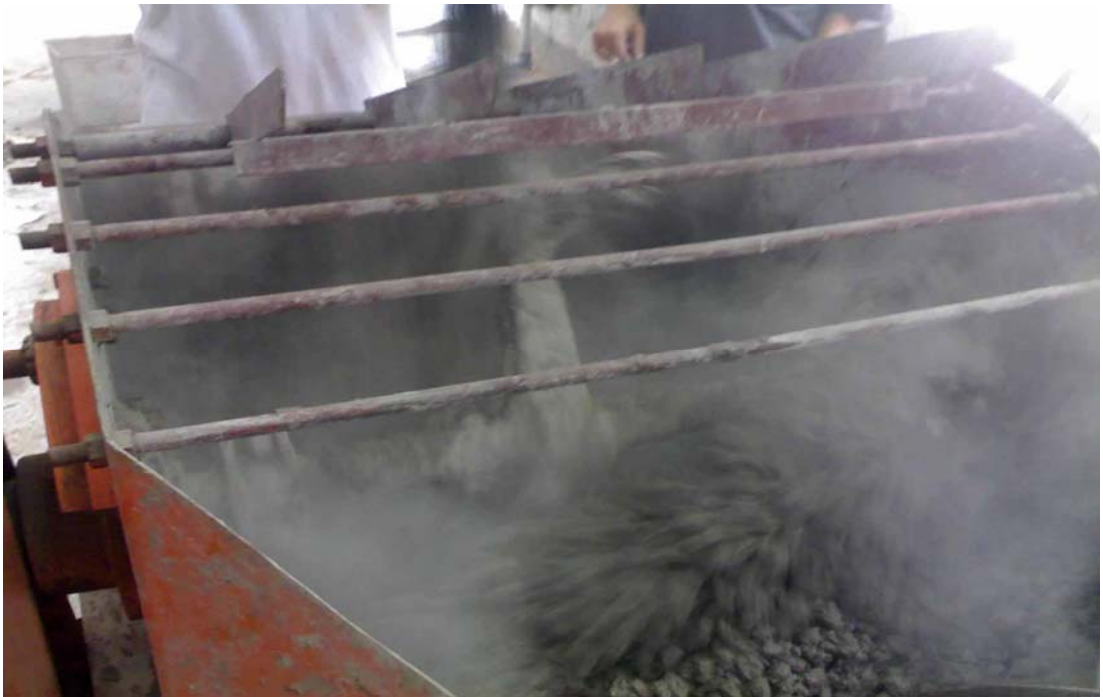
Fig.3.4: Pouring of aggregate in mixer machine
