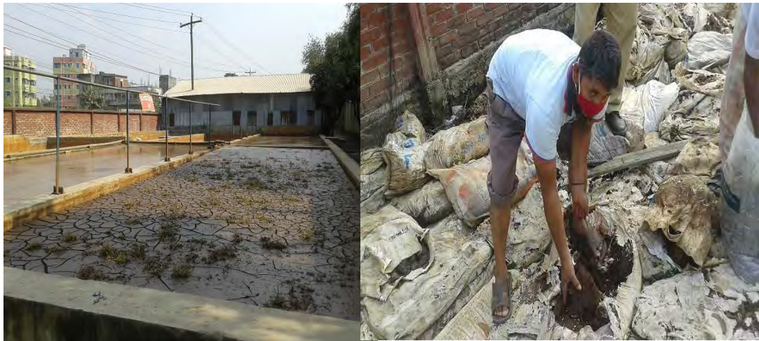
Figure 3.2. Raw sludge pond and stabilized bed (dump site)
