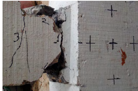
Fig. 5.8: Disintegrate the concrete
