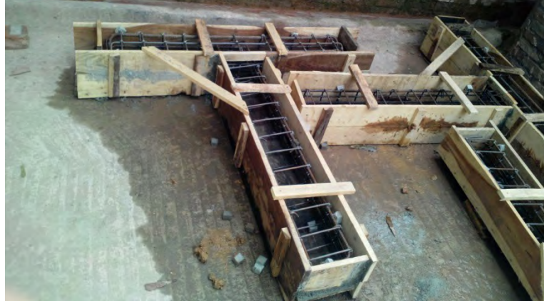
Fig. 4.5: Preparation of Formwork
