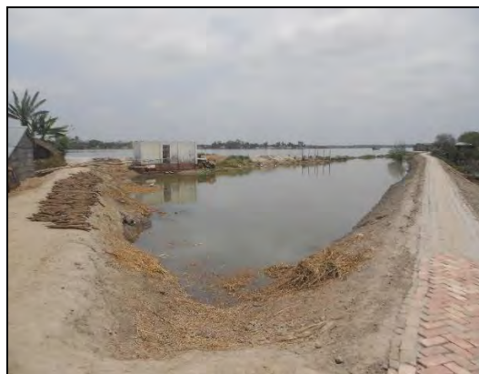
Photo B2: Ring embankments undergoing rehabilitation after Aila.
