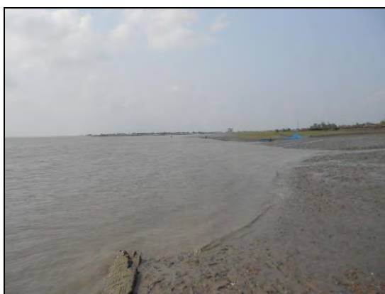
Photo B3: Breaching caused by Aila at Nalian sluice.
