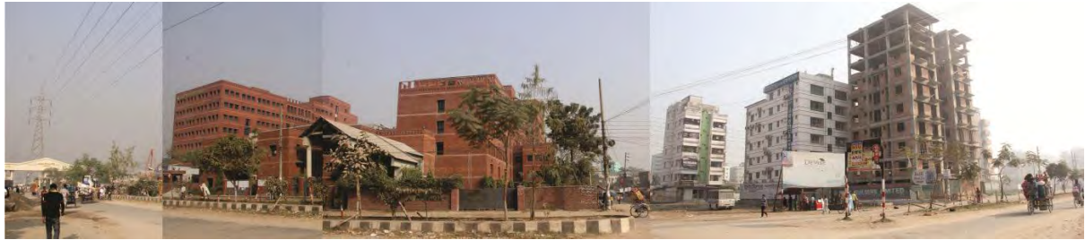
Figure 3-20 Site Surroundings in reality from south
