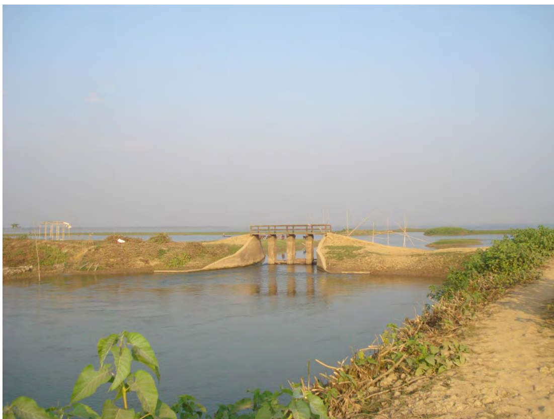
Photo 8.1 Drainage of water through Ghatia regulator
