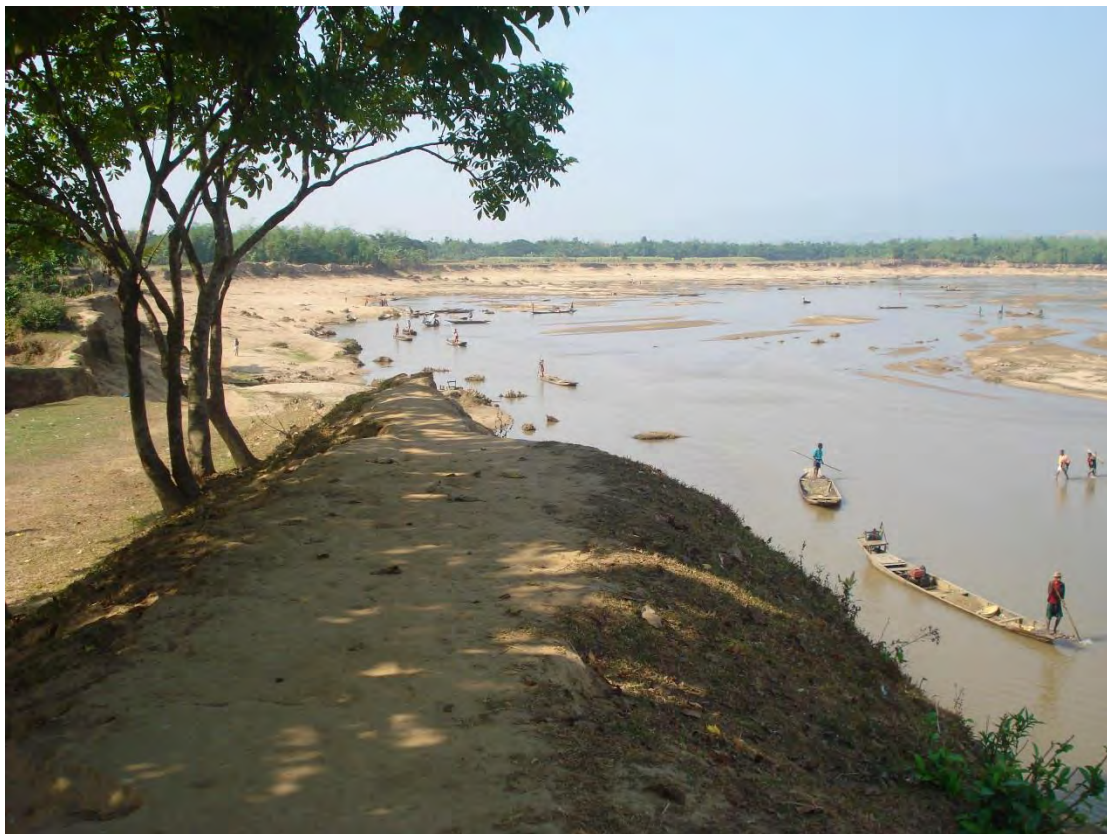
Photo 5.2 Damaged embankment at Adang village
