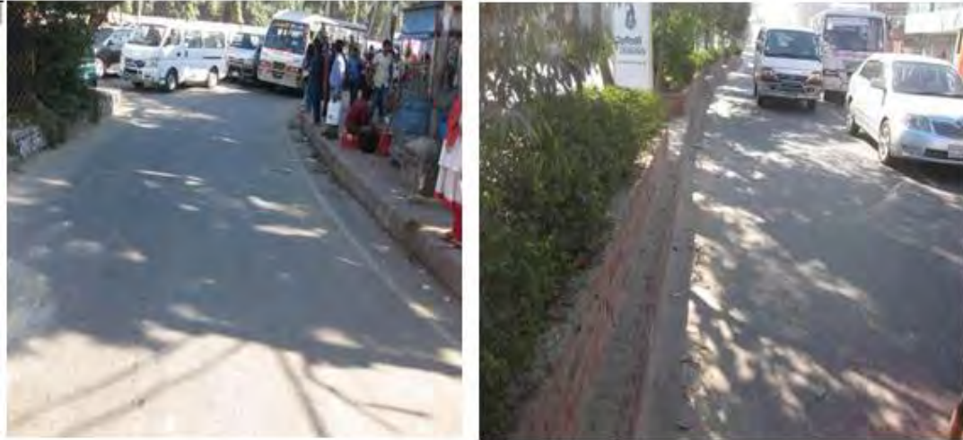
Figure 1.2.4: Inside the Intersection: (a) Left Turning Lane and (b) Right Turning Lane.
