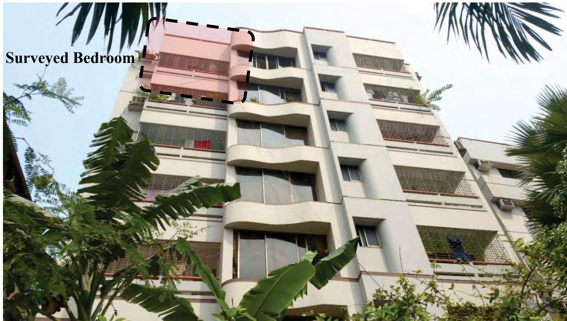
Fig. 4.5: Image of the Surveyed Building
