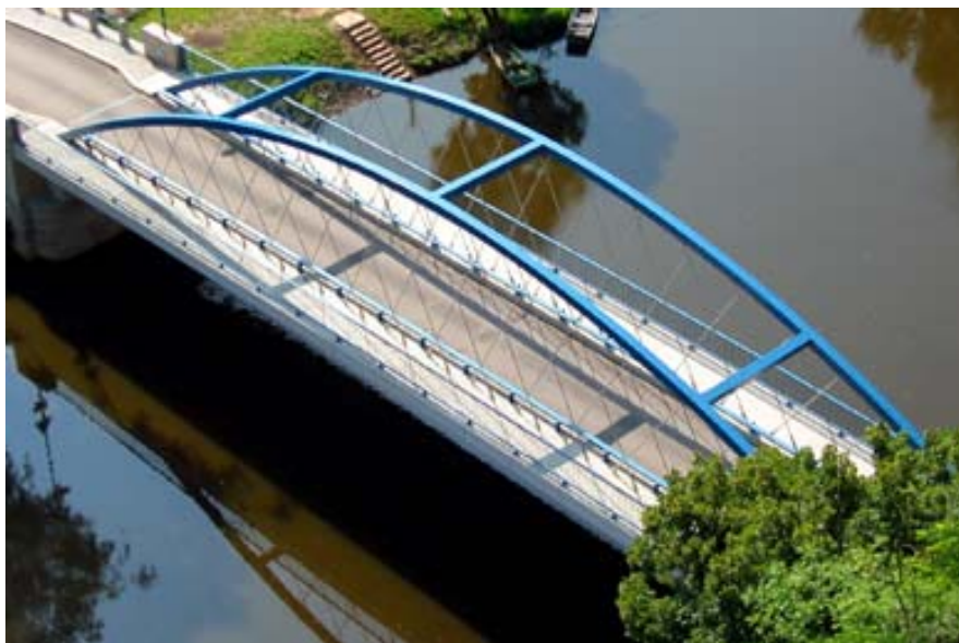
Figure 5.1: Network Arch Bridge in Czech Republic Opened to Road Traffic in 2004 [8]
