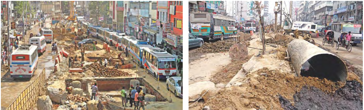
Fig 5.3 & 5.4: Condition of walkway in Maghbazar
