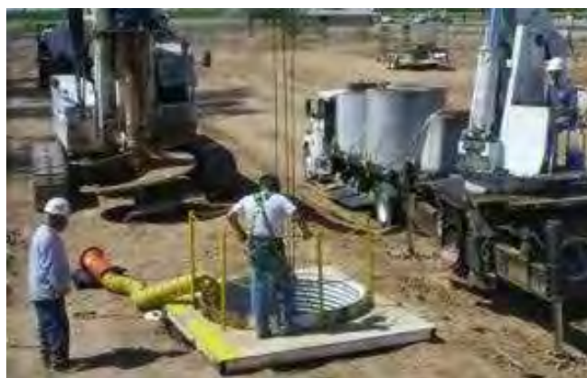
Fig - 4.2 Job Site Safety - Basic Drilling Co. [11];
