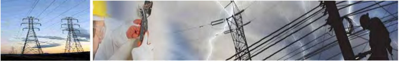
Fig-3.18 Electrical Hazards [48];
