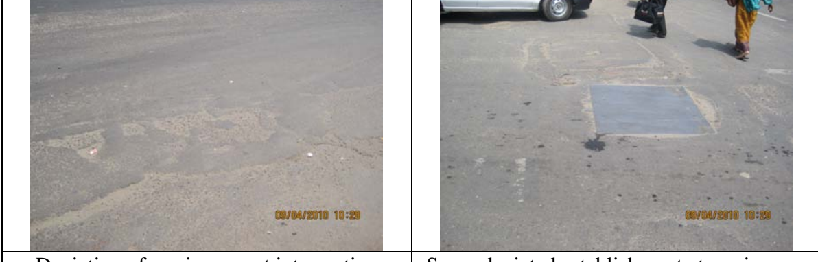
Deviation of carrigeway at intersection
