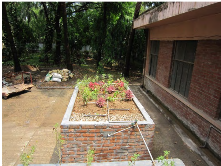
Figure 13: Vegetation in subsurface flow constructed wetland.
