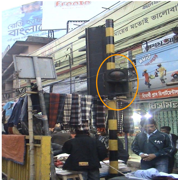
Figure 4.25a) Pedestrian Signal Head Condition in Palton(Topkhana)
