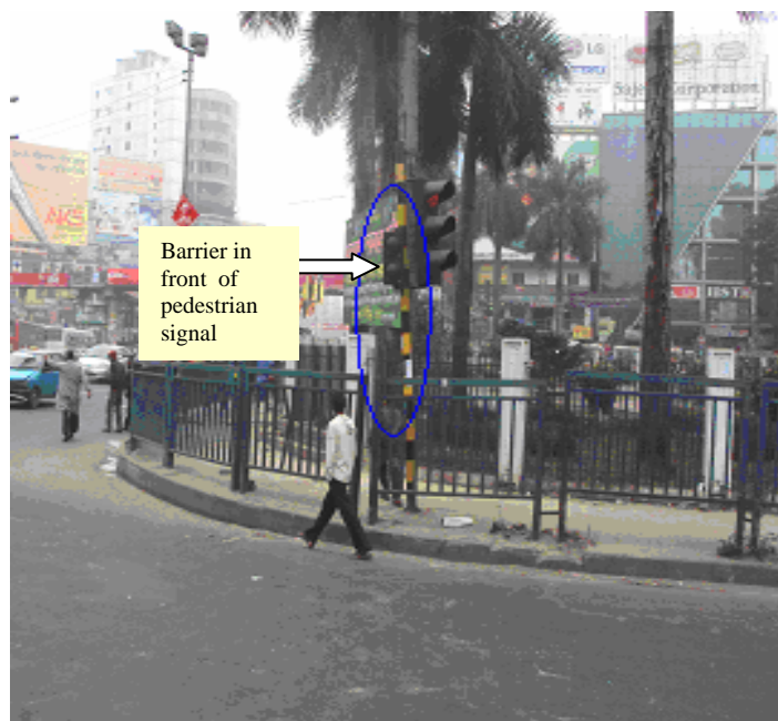
Figure 4.22: Pedestrian Signal Pole Positioning is Wrong at West Approach in Farm Gate Intersection.
