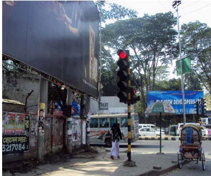
Figure 31c): Sight distance is restricted due to Bill board in left sight at Matshaw Bhaban
