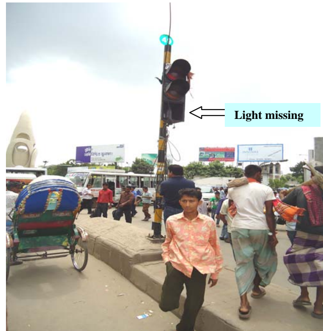
Figure 4.4 b: Signal Light Condition in Gulistan Square Intersection
