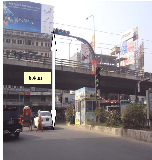
Figure 4.15 b) Signal Head Assembly in Mast arm at Mohakhali Amtoli Intersection
