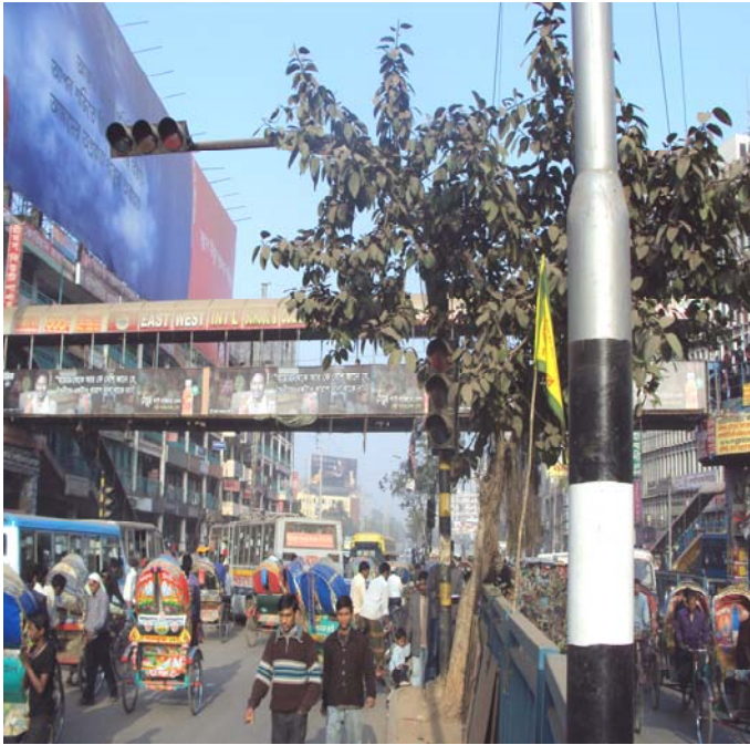
Figure 4.38a): Signal Light Condition in Mirpur 1 Intersection.
