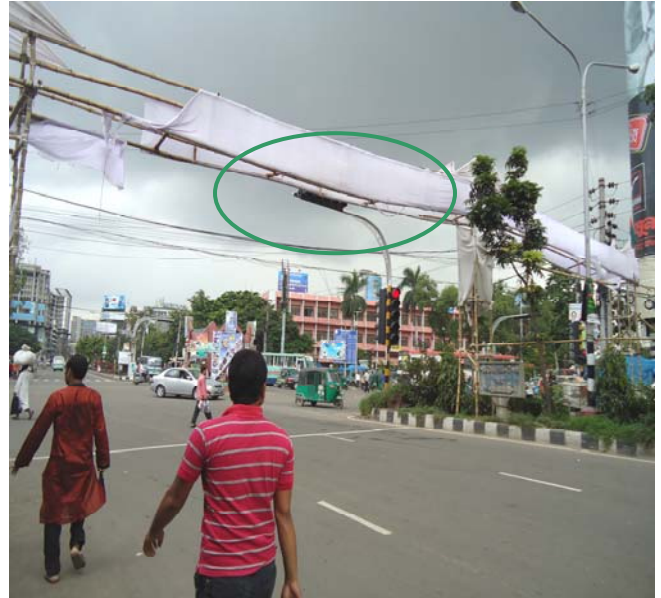
Figure 10: Signal Light is not Visible at Mast Arm in Zero point Intersection
