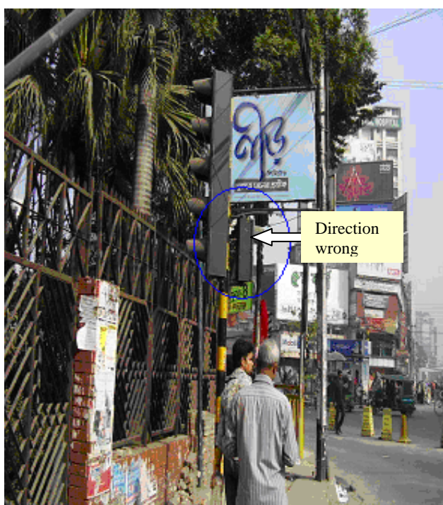
Figure 4.24 a) Pedestrian Signal Face is not to the Direction of the Traffic flow at Kakrail
