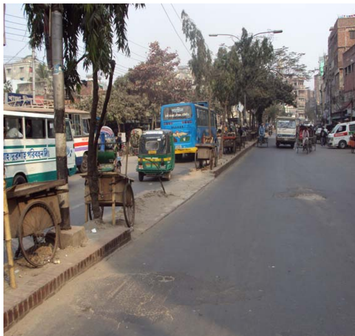
Figure 4.29: Median Condition at East Approach in Dholaikhal Intersection.
