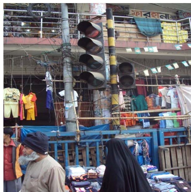
Figure 4.11b): Access Condition for Maintenance of Signal Zahir Raihan Intersection.
