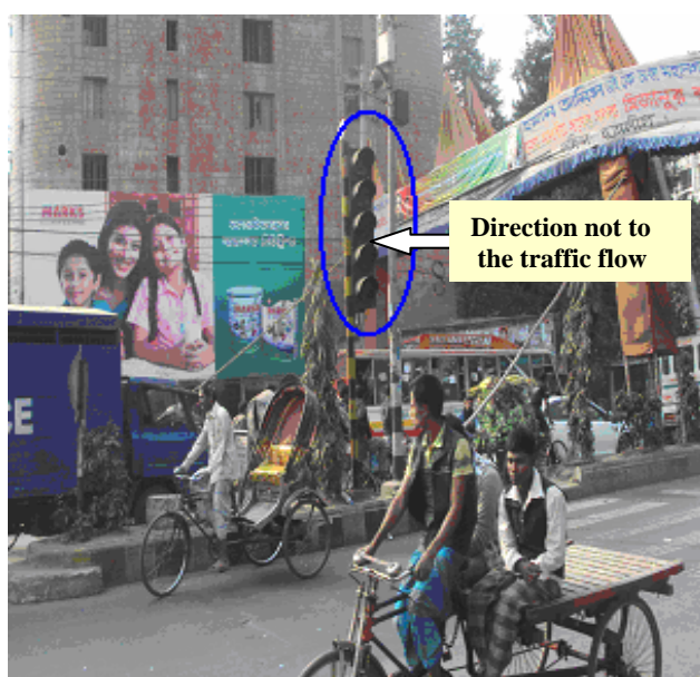
Figure 4.14a) Signal Head Direction Wrong at North Approach in Sadarghat Intersection.
