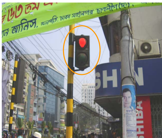
Figure 26: Pedestrian Signal Face is not Clear at Bijoyagar Intersection
