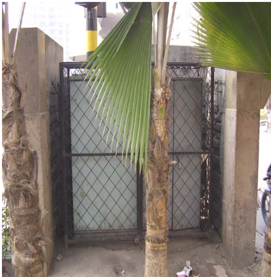
Figure 4.5 a: Access Condition of Signal Controller Cabinet at Bijohnagar Intersection.
