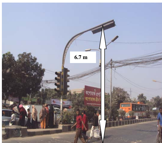
Figure 4.6: Mast arm Height at North Approach of Natun Bazar inetersection
