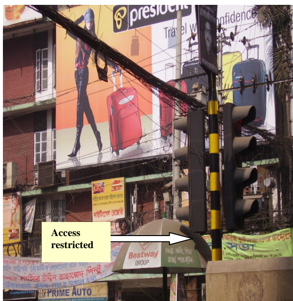
Figure 4.11a): Access Condition for Maintenance of Signal at South Approach in Bijoy Nagar
