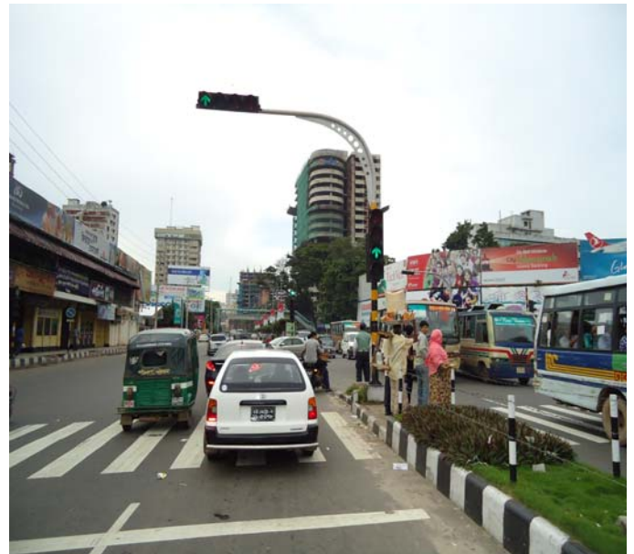
Figure16: Wrong Placement of Signal at Hotel Sheraton Interspersion
