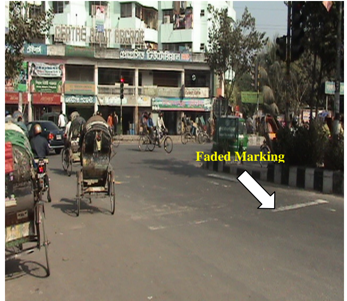
Figure 4.18d) Faded Marking in Pirjangimazar Intersection
