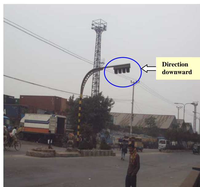
Figure 4.14 b) Signal Head Direction is not Towards the Flow of Traffic in Kamalapur Container
