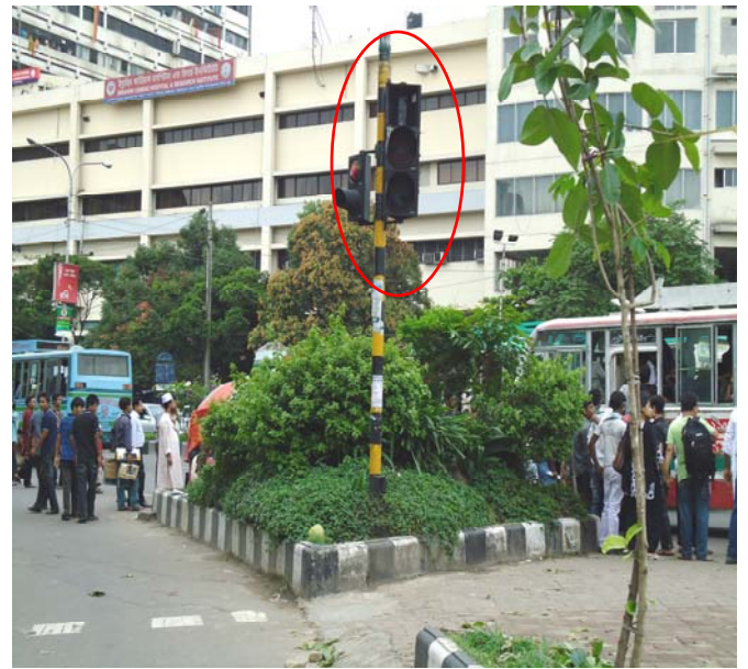
Figure 14: Signal Light Broken in Shahbagh Intersection
