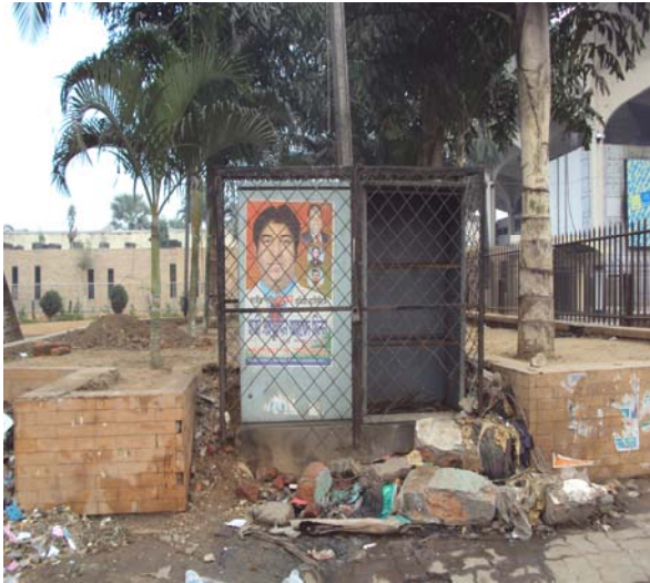
Figure 4.5 c: Signal Controller Cabinet Condition at Kamalapur Station.
