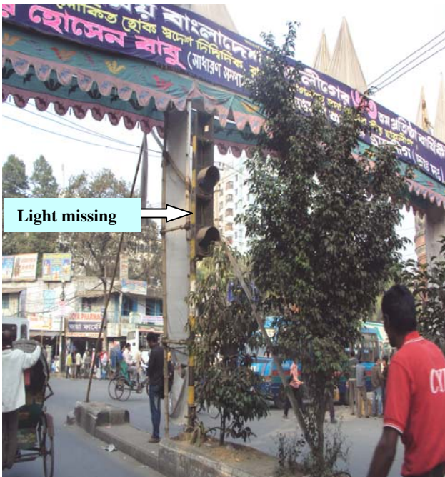
Figure 4.4 a: Signal Light Condition at South Approach in Sadarghate Intersection.
