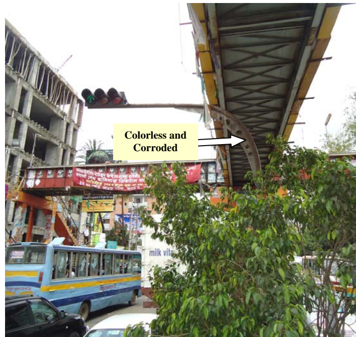
Figure 4.7: Mast Arm Condition in Science Lab Intersection.
