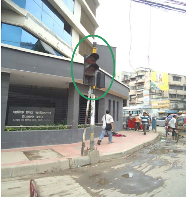
Figure 5: Signal Head Broken in Ittefaq Intersection
