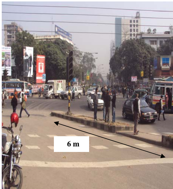
Figure 4.2 a: Placement of Traffic Signal in Banani Kakoli Intersection.
