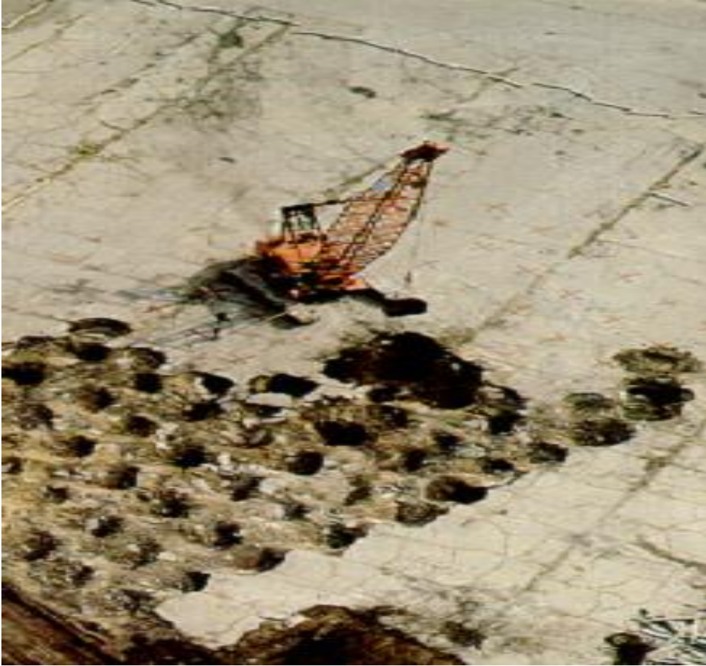
Fig 2.13: Photograph showing dynamic compaction technique
