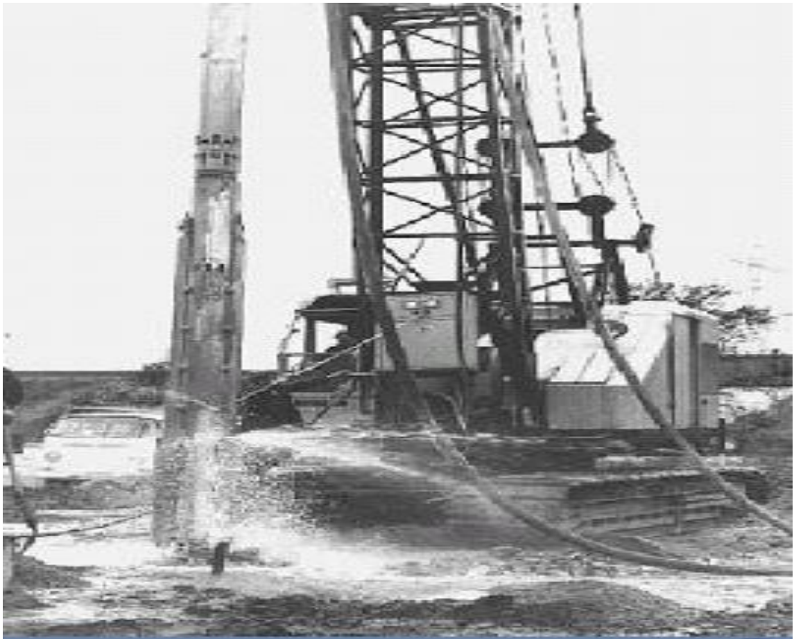
Fig 2.12: Photograph showing Vibroflotation technique
