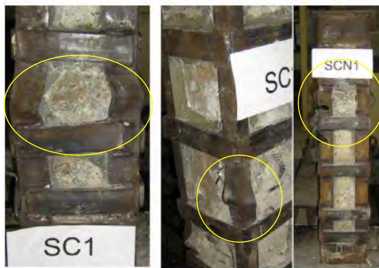
Figure 2.4 Failure modes of jacketed columns with buckling of corner angle
