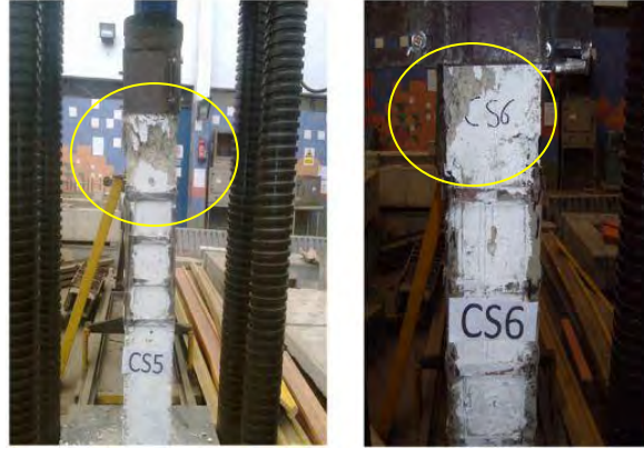
Figure 2.5 Failure at un-strengthened part of partially jacketed columns
