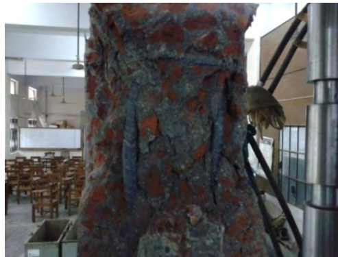
Figure 5.5 Buckling of longitudinal reinforcements in un-strengthened RC column under concentric loads
