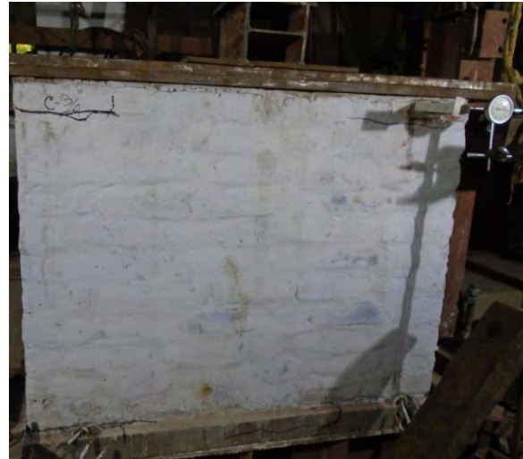
Figure 4.27 Final Crack Pattern of Specimen C-3/4
