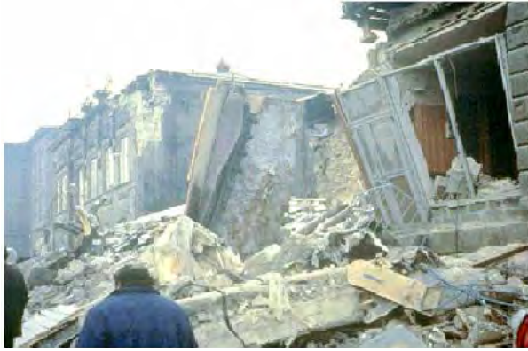
(a) Armenia earthquake December 7, 1988
