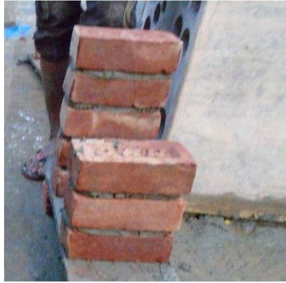
d. Construction of clay burnt brick with mortar thickness 3/4".
