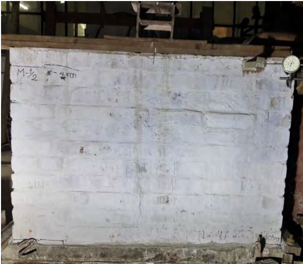
Figure 4.32 2 nd and 3 rd Cracks Patterns of Specimen M-1/2
