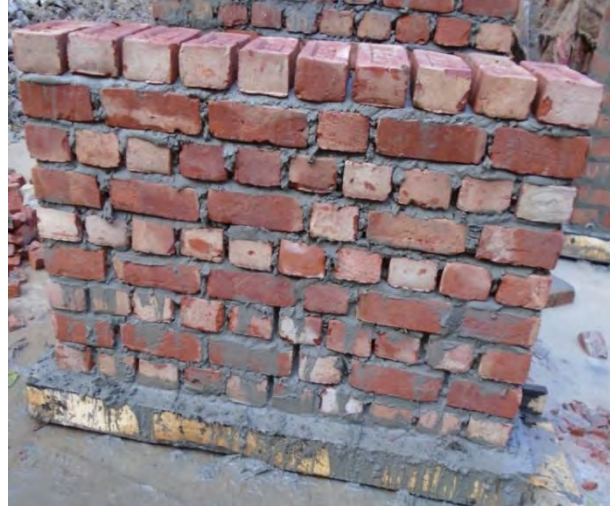
d. Construction of clay burnt brick wall with 3/4" mortar thickness
