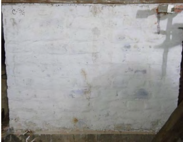
Figure 4.24 Initial Crack (Flexure) Patterns at Base of Specimen C-3/4
