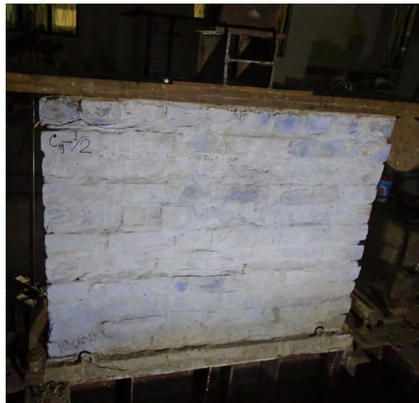
Figure 4.21 2 nd Crack (Shear) Pattern of Specimen C1-1/2
