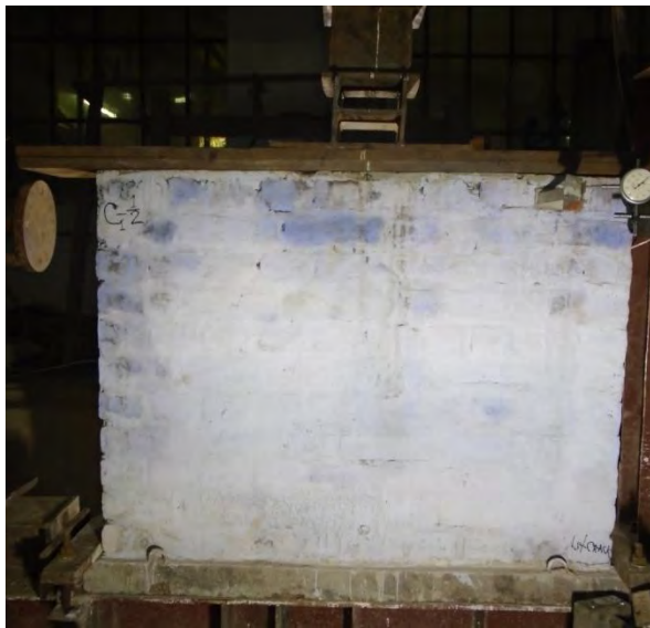
Figure 4.20 Initial Crack (Flexure) Pattern of Specimen C1-1/2
