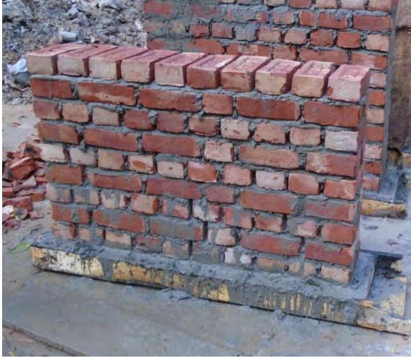
c. Construction of clay burnt brick wall with 1/2" mortar thickness
