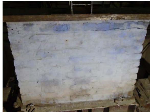
Figure 4.18 2 nd Crack (Shear) Pattern of Specimen C-1/2
