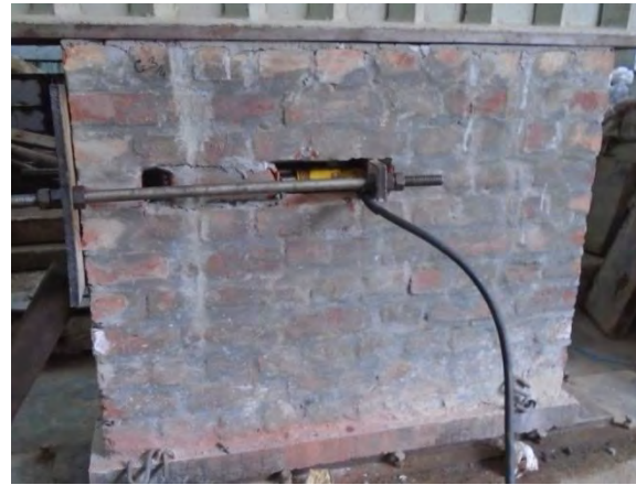
Figure 4.12 Failure pattern of shear test specimen C1-3/4
