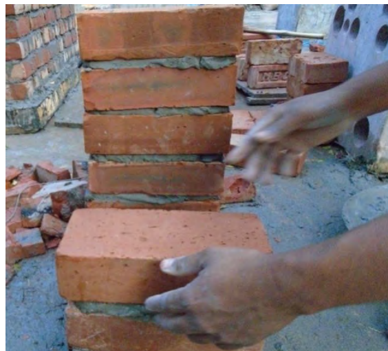
b. Construction of machine made prism with mortar thickness 3/4".
