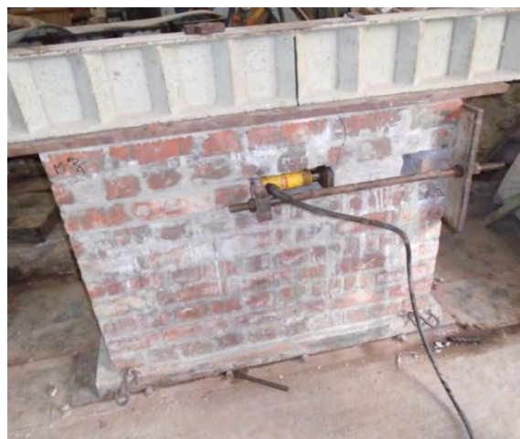
Figure 4.15 Failure Pattern of Shear Test Specimen M-3/4
