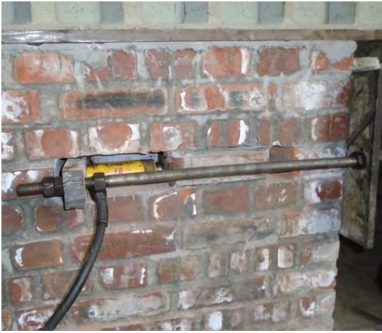
Figure 4.13 Failure Pattern of Shear Test
