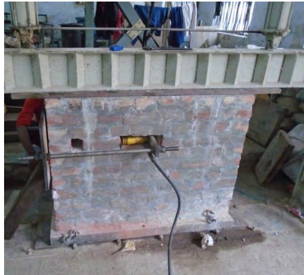
d. Shear test setup of clay burnt brick wall (C1-3/4) with mortar thickness 3/4"
