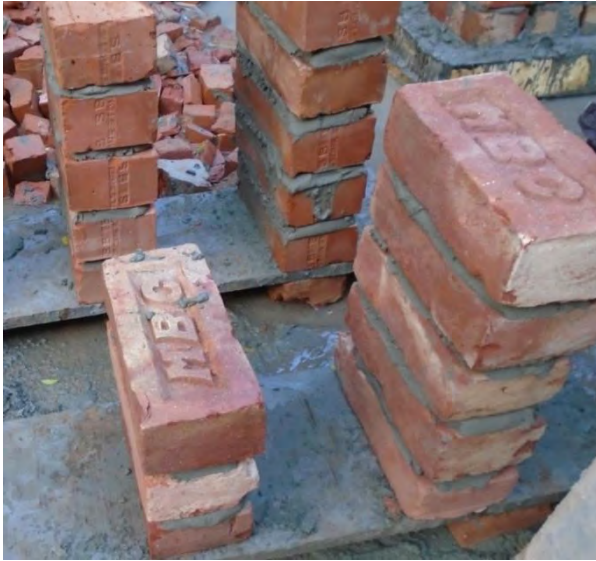
c. Construction of clay burnt brick prism with mortar thickness 1/2".
