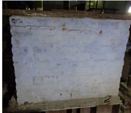
Figure 4.29 2 nd Cracks (Shear) Patterns of Specimen C1-3/4
