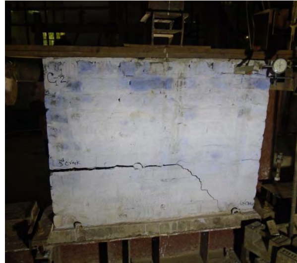
Figure 4.23 Final Crack Pattern of Specimen C1-1/2
