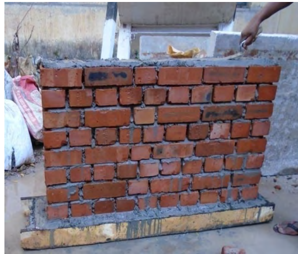
b. Construction of machine made brick wall with 3/4" mortar thickness
