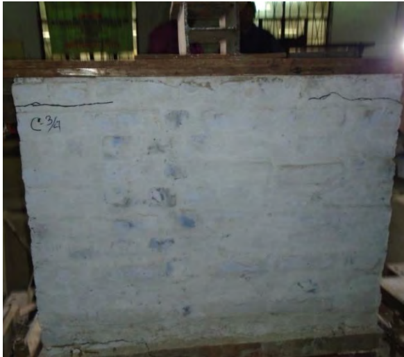
Figure 4.26 3 rd Cracks (Shear) Patterns of Specimen C-3/4
