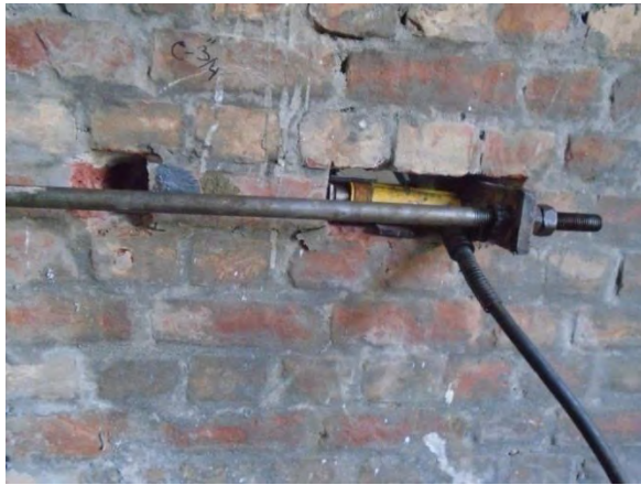
Figure 4.11 Failure pattern of shear test Specimen C-3/4
