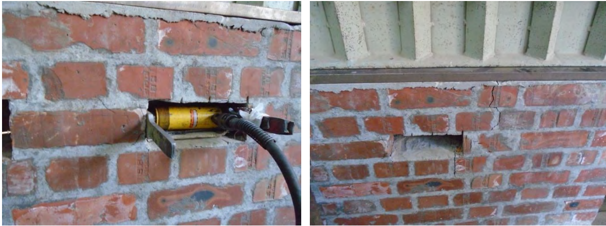
Figure 4.16 Failure Pattern of Shear Test Specimen M1-3/4
