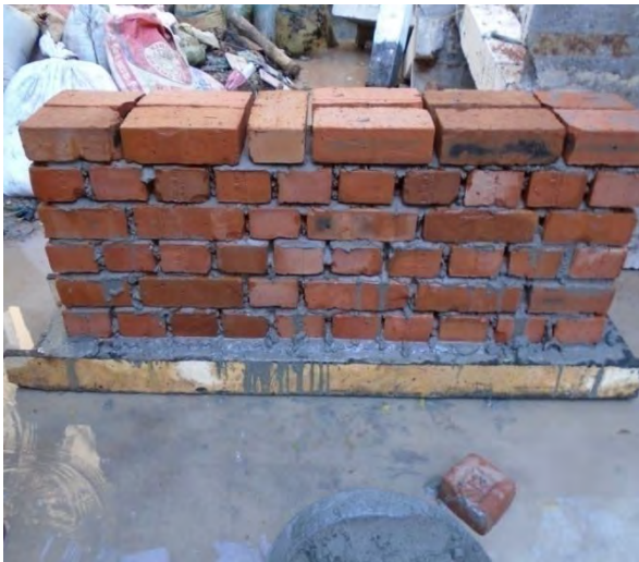
a. Construction of machine made brick wall with 1/2" mortar thickness
