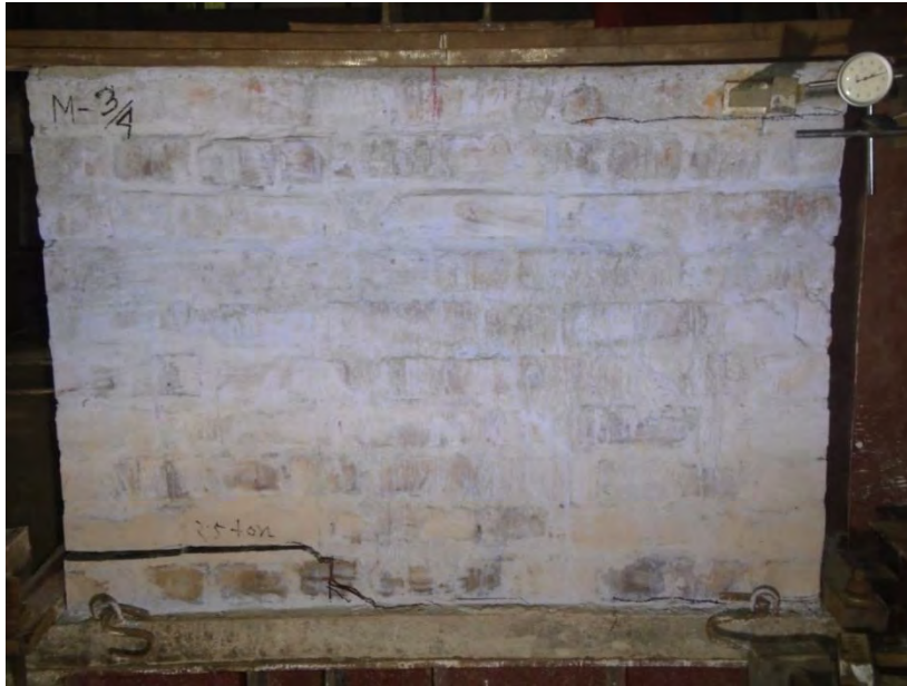
Figure 4.39 Final Crack Pattern of Specimen M-3/4
