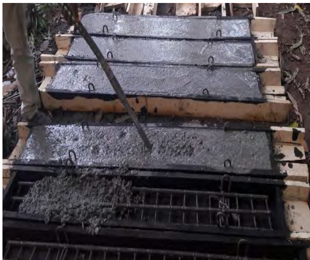
Figure 3.4: Compaction of Fresh Concrete into Formwork using Vibrator
