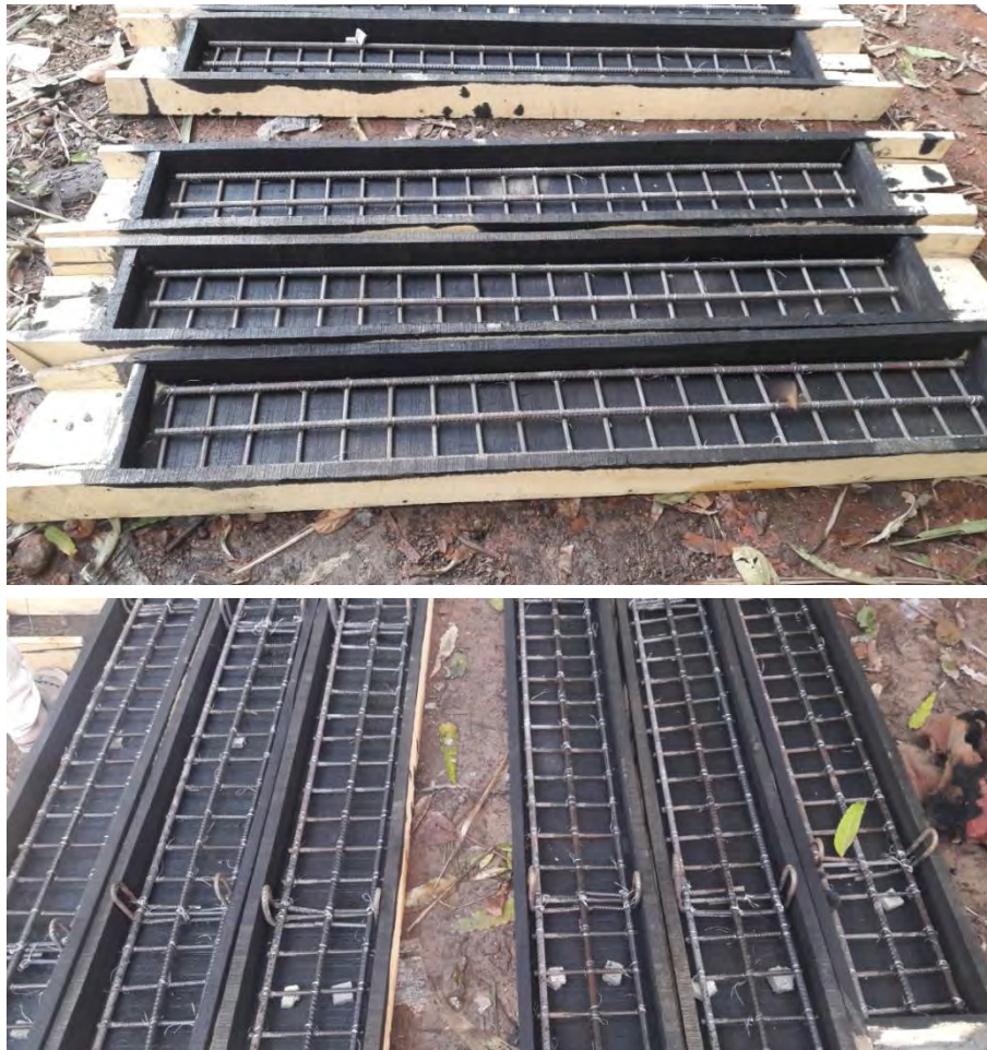
Figure 3.3 Reinforcement Placement on formwork
