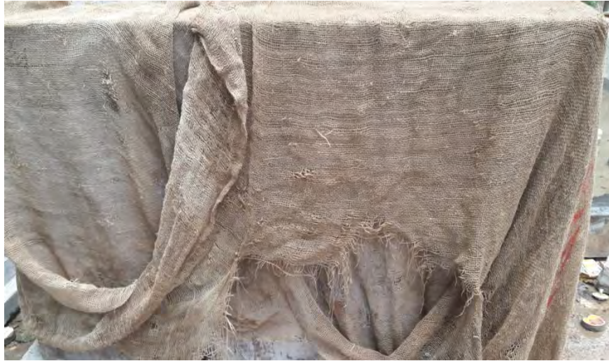
Figure 3.6 Curing of Sample
