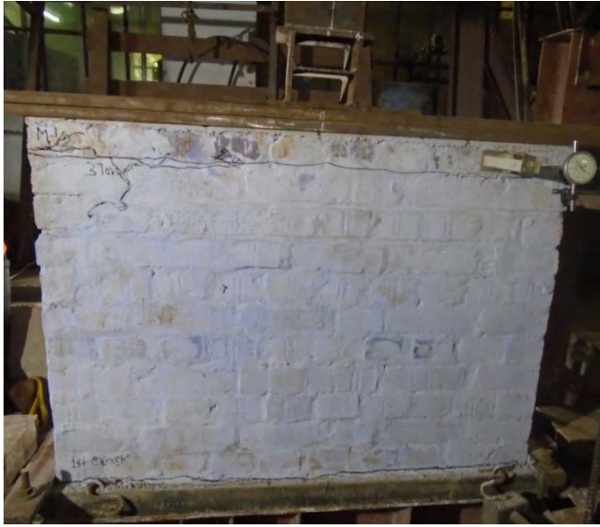
Figure 4.36 Final Crack Pattern of Specimen M1-1/2
