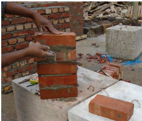
a. Construction of machine made prism with mortar thickness 1/2".
