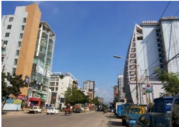
Figure 4.8: Emerging high rise commercial buildings along the secondary street of Uttara
