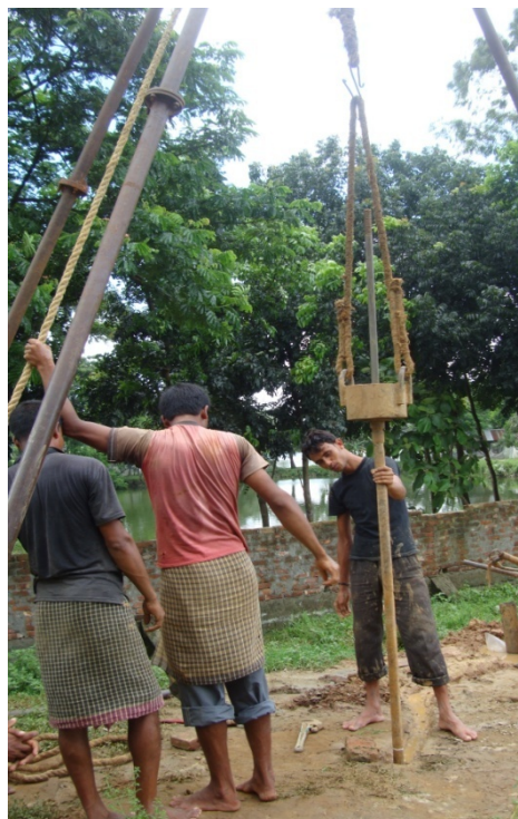
Fig. 3.3: SPT hammer release arrangement
