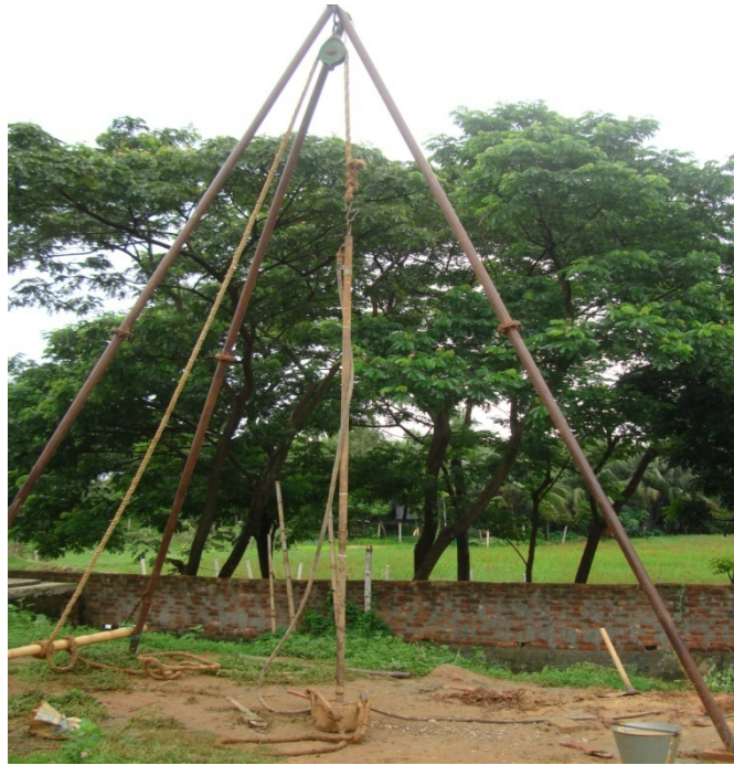
Fig. 3.2: Arrangement for performing Wash boring
