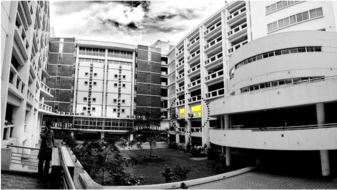
Figure 3.16: 2 nd floor view (Circled) of AUST architecture department.
